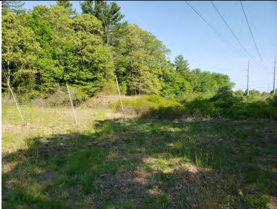
Photo 5: View of the existing TNEC transmission ROW at the TNEC Davisville Transmission Tap Lines. The TNEC ROW will be widened to accommodate new overhead lines from the ICF to the TNEC Davisville Substation and from the ICF to the TNEC Davisville Transmission Tap. Photo date: May 20, 2021
