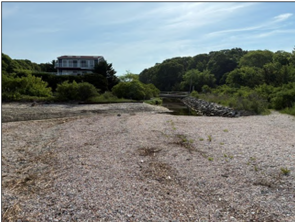
Photo 4: View of Mussachuck Creek Inlet. Standing on the main plug of material. (Facing the Nayatt Rd. Bridge to the East)
