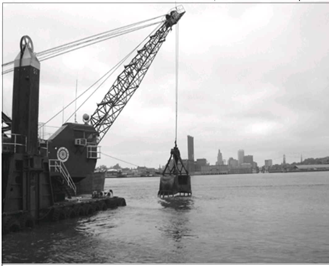
A gaping clam shell bucket is lowered to the bottom of the Providence River to scoop out a load of sediment as part of the Providence River and Harbor Dredging Project. The project will restore the seven-mile long Providence River Shipping Channel to its federally mandated 40 foot depth and 600 foot width.
