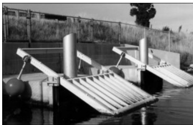
Tidegates at the Galilee Salt Marsh restoration site open to flood a restored salt marsh that had been destroyed after a road was built and blocked the twice-daily tides from reaching the marsh.
