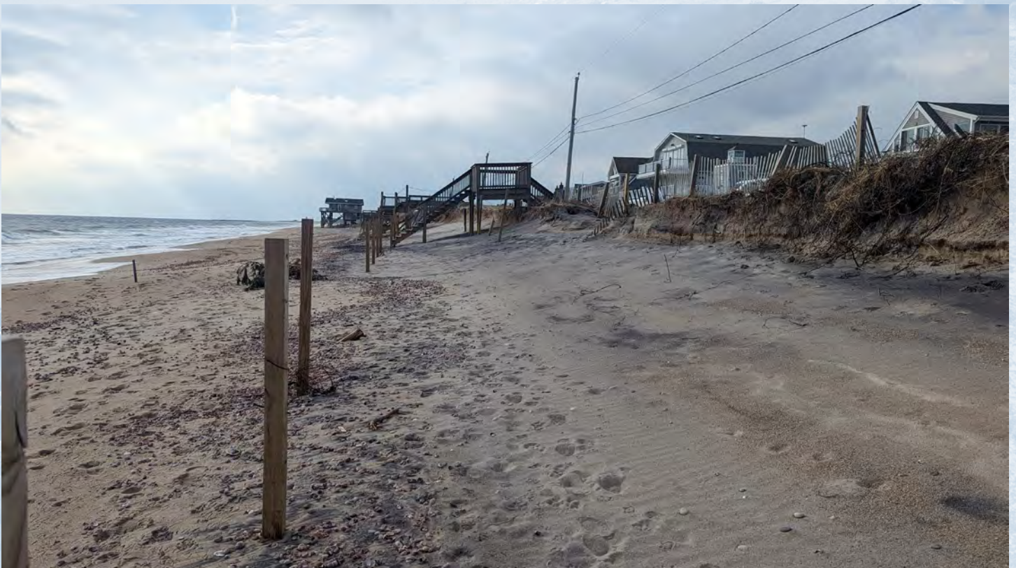
Charlestown Beach Road, South Kingstown
