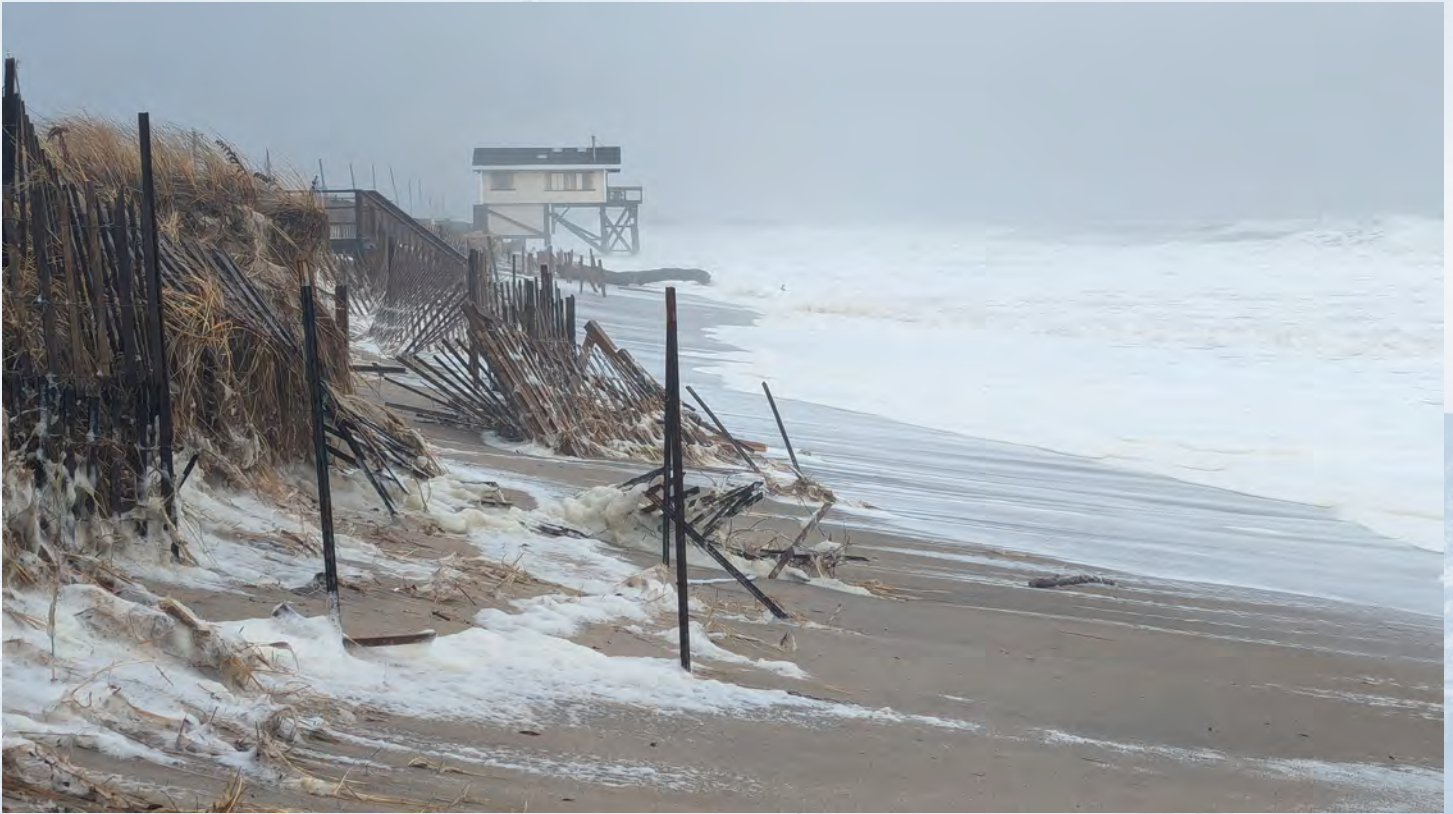
Charlestown Beach Road, South Kingstown
