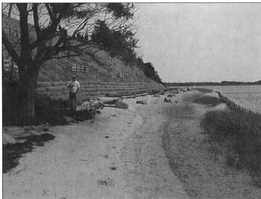
Figure 2B. The same coastal bank/bluff as shown in figure 2A showing a coir fiber roll revetment, that is, non-structural coastal armoring, that is preventing sand from eroding from the bank and feeding the fronting and adjacent beach and dunes.
