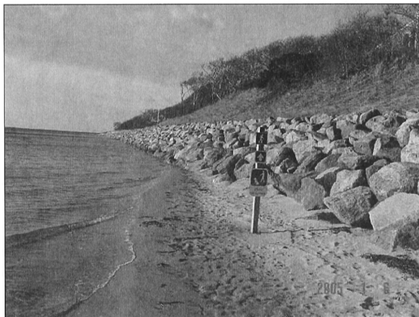
Figure 7. The loss of public lateral beach access due to shoreline armoring along the shore of Chatham, Massachusetts. Prior to revetment construction, a dry sandy beach provided lateral public beach access to a U.S. Fish and Wildlife property.
