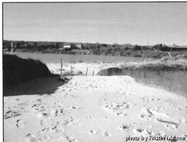
Ocean has broken through dune to pond side.
