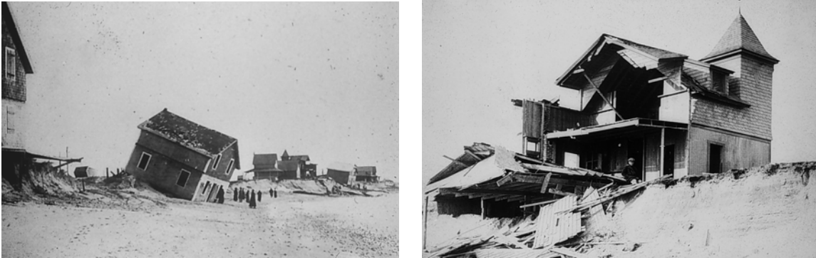
Storm erosion and destruction – 1900
