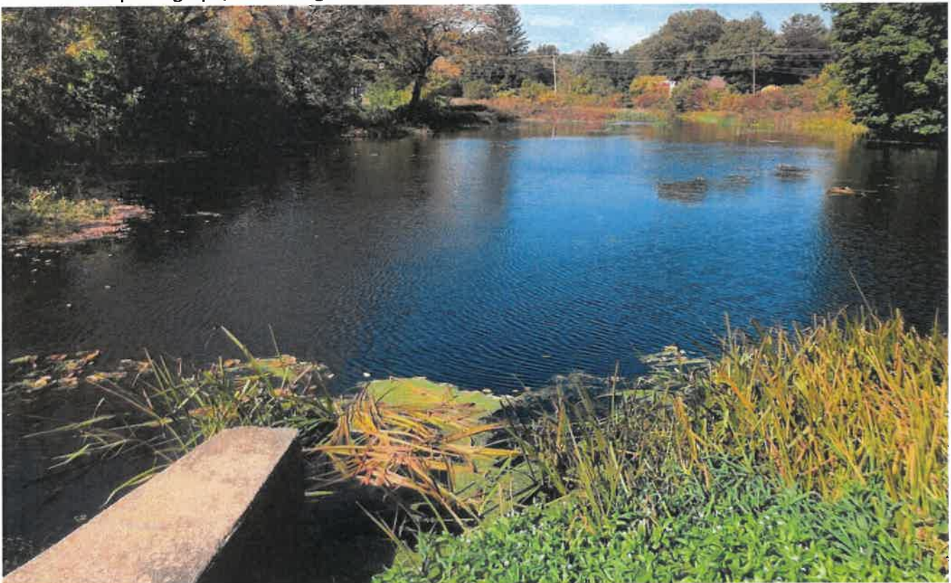
Figure 3: View northwest of the impoundment looking upstream from the dam structure. Photo taken November 8, 2022.
