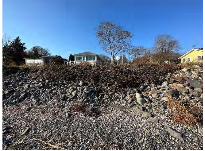
Photo 2. West view of the deteriorating Coastal Bluff east of Edda Avenue. The existing scattered stone will be removed prior to the construction of a riprap revetment.
