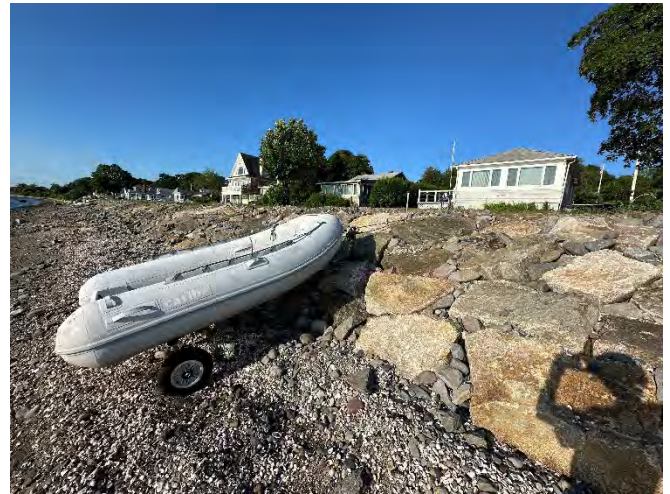
Photo 7. Southwest view of the partially constructed stone revetment east of Edda Avenue, appearing as a close-up of Photo 6. Note how the revetment stone has been placed and set at an unobtrusive low profile.
