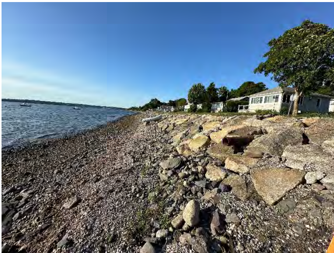
Photo 6. South view of the partially constructed stone revetment and unvegetated coastal Beach east of Edda Avenue, at northern limit of Project. Note how the beach ramp/fringe has remained intact. The completed revetment will extend from Edda Avenue southward to Alice Avenue.
