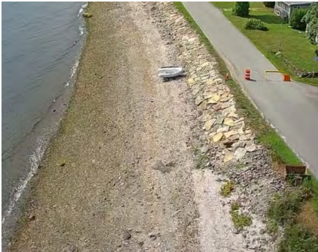
Photo 9. Drone imagery showing south view of the completed revetment at the north end of the Project, opposite Edda Avenue. Portions of the Bluff not subject to the Project are visible in the foreground for comparison.
