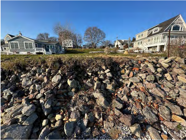
Photo 1. West view of the deteriorating Coastal Bluff east of Madison Avenue. Structural shoreline protection in the form of a riprap revetment will be constructed to reinforce the Bluff and prevent further erosion.
