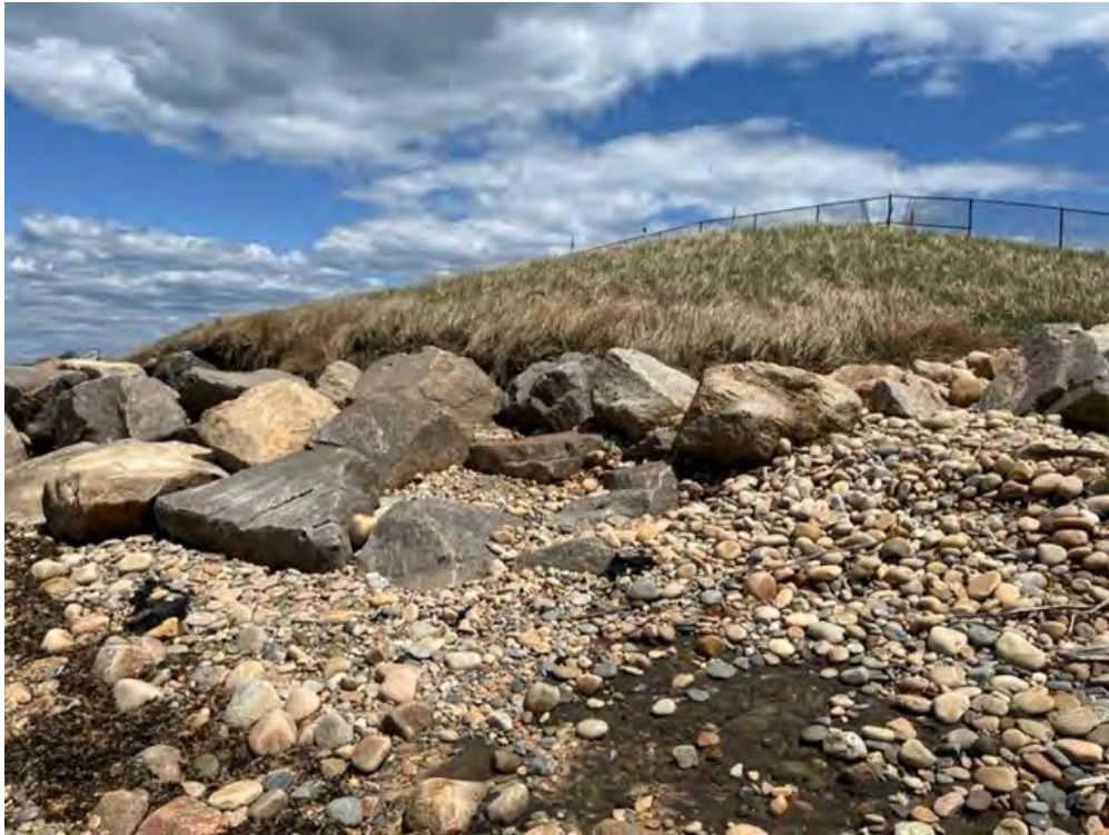
Photo 3: Overview of south corner of landfill slope at shoreline – note cobble wash into revetment and erosion/scarp above revetment
