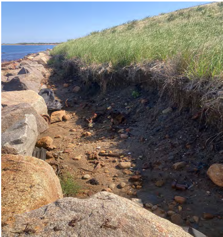
Photo 10: Erosion of earth slope and vegetation above revetment stone caused by storm waves
