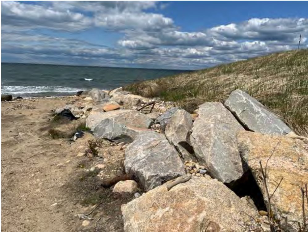
Photo 5: Note erosion and possible revetment stone movement caused by storm waves
