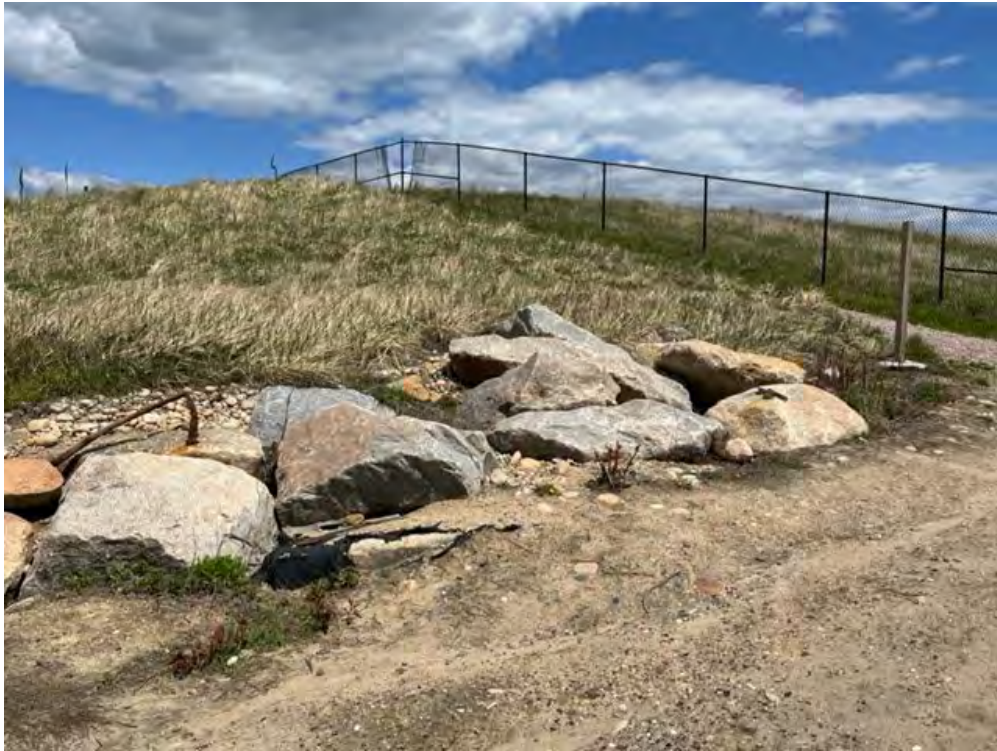
Photo 1: Overview of south end of the landfill slope - note erosion behind revetment
