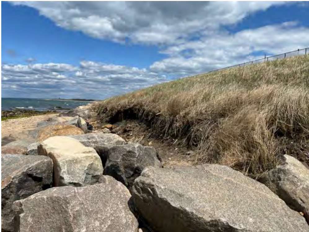
Photo 4: Note erosion/scarp behind revetment stone caused by storm waves
