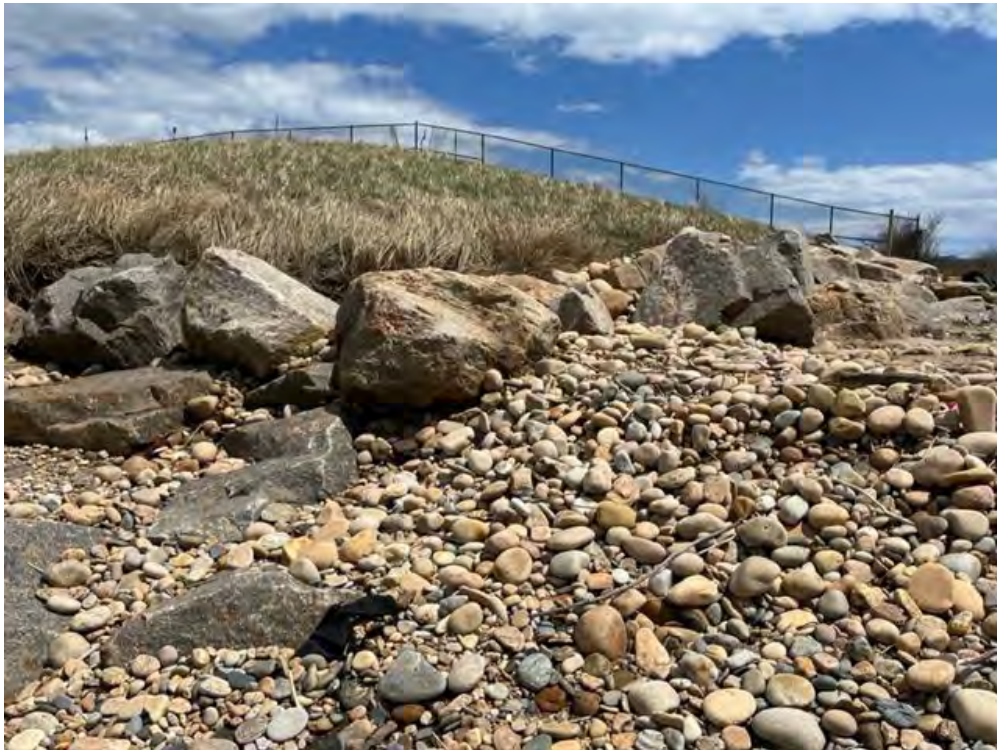
Photo 6: Overview of south corner of landfill slope at shoreline – note cobble wash into revetment and erosion/scarp above revetment
