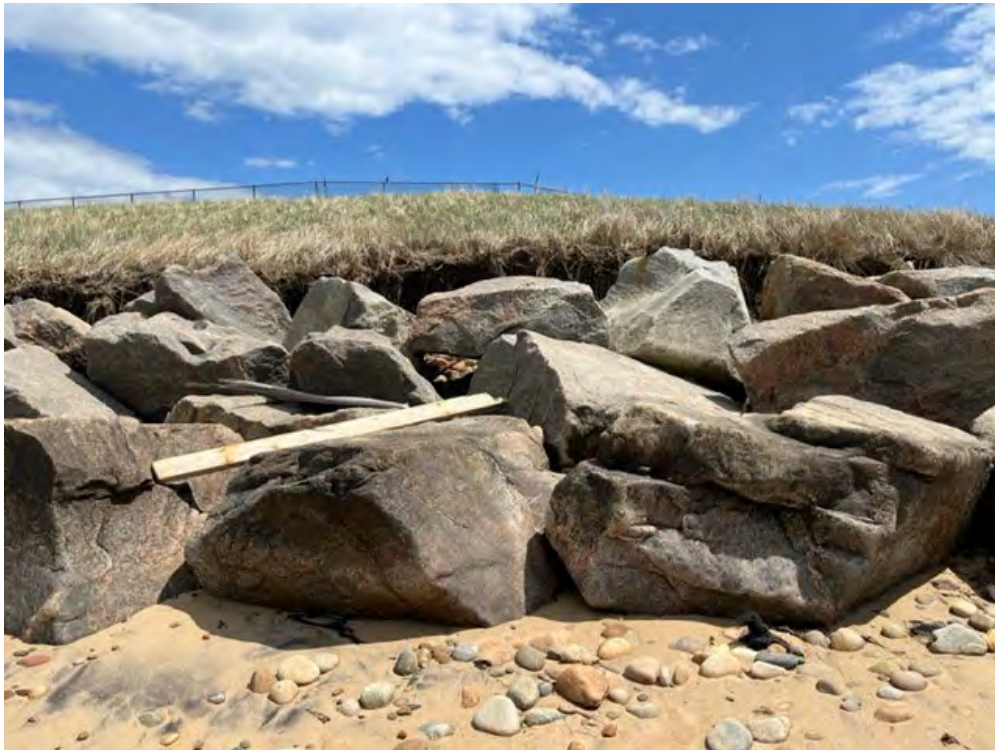
Photo 8: Overview of revetment stone – note erosion/scarp behind revetment caused by storm waves
