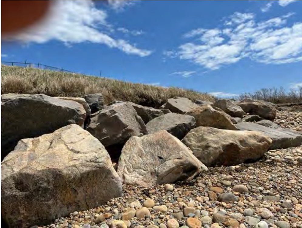
Photo 7: Typical revetment toe stone section
