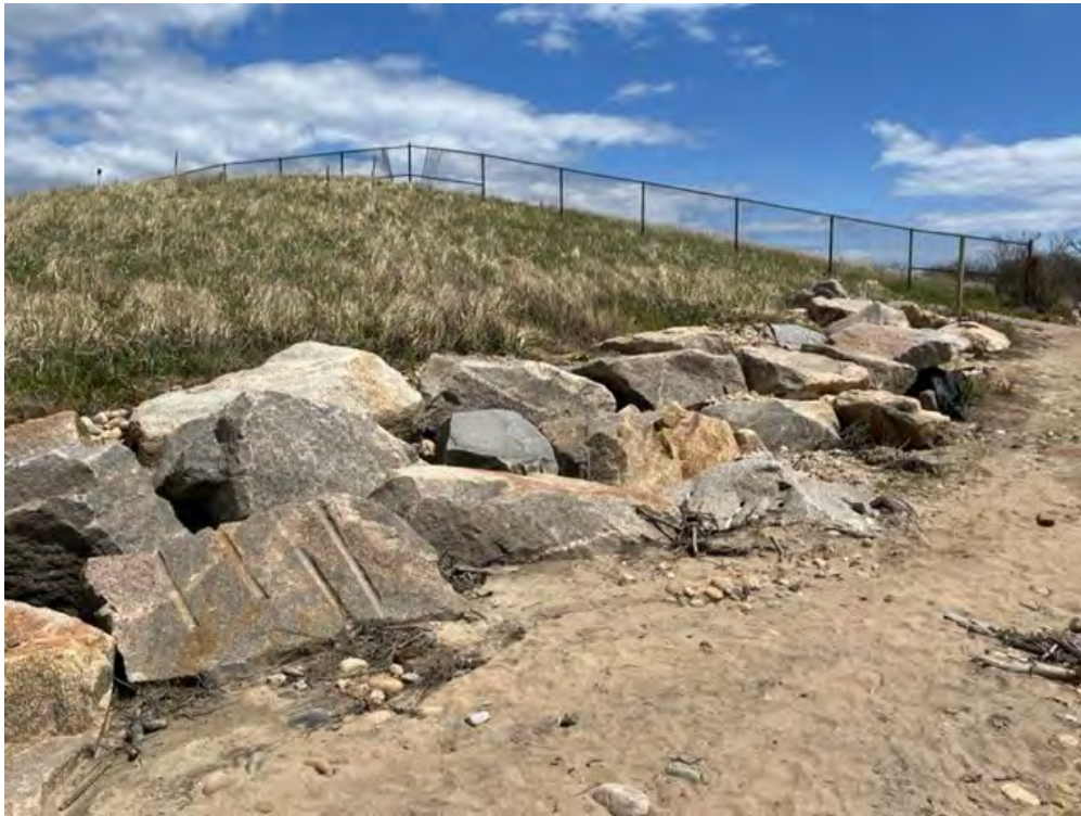
Photo 2: Overview of south end of landfill slope – note erosion/scarp behind revetment
