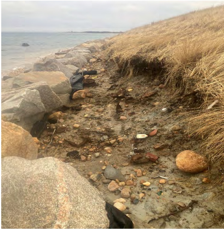
Photo 9: Erosion of earth slope and vegetation above revetment stone caused by storm waves
