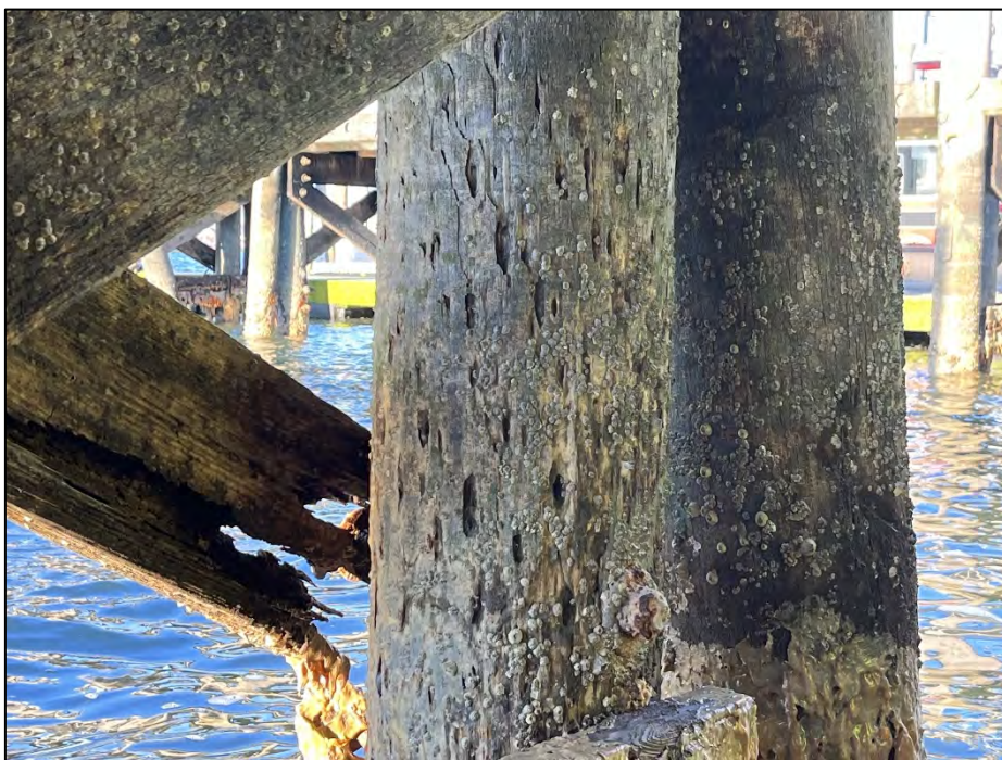
Photo No. 3.: Typical deterioration of pile and cross bracing on Pier "G".
