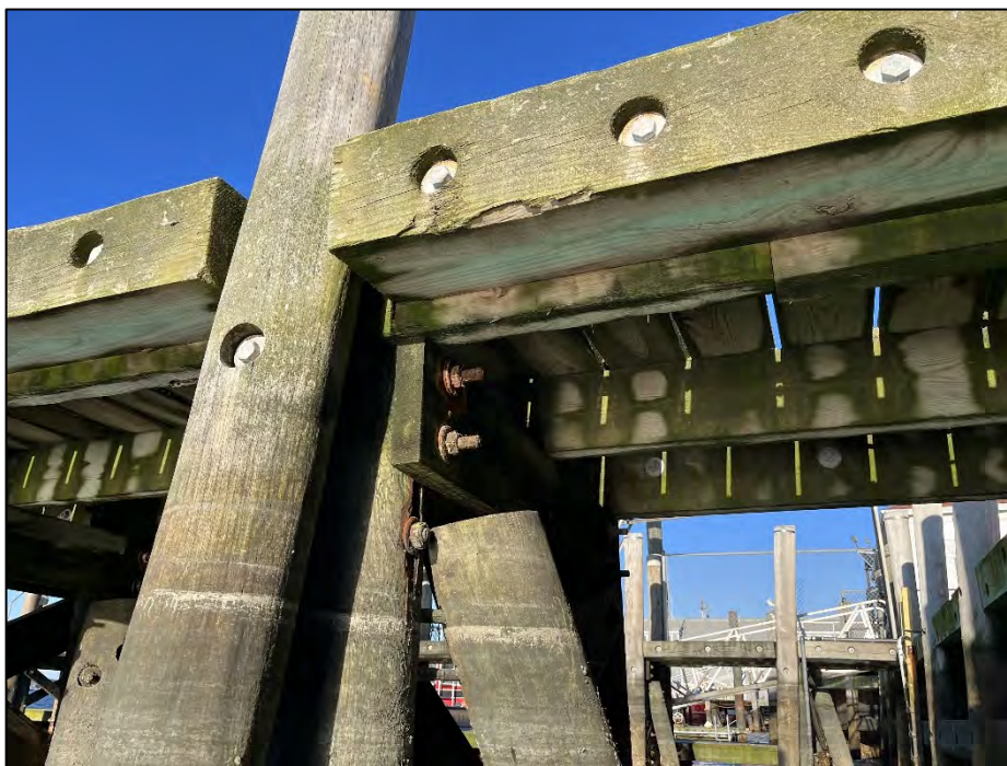
Photo No. 5.: Weathered timber below the decking of Pier "G".
