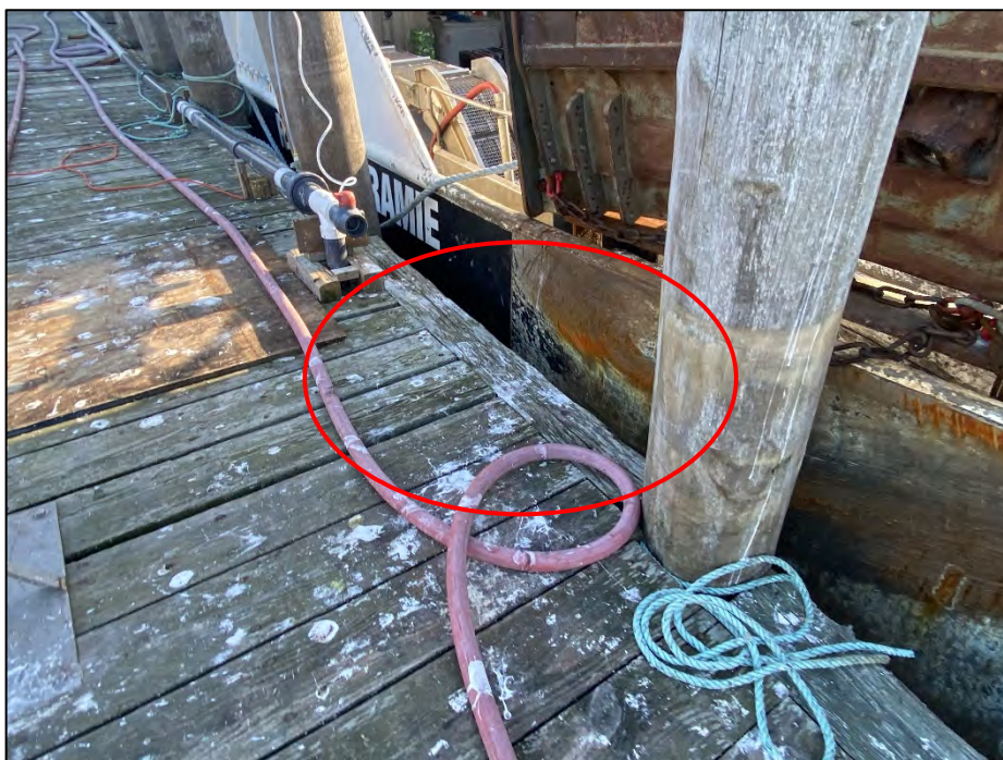
Photo No. 4.: Deterioration of timber chocks typical of Pier "G".
