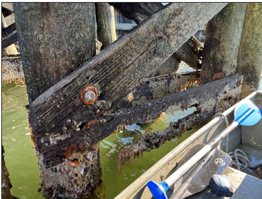
Photo No. 2.: Typical deterioration of pile and cross bracing on Pier "G".
