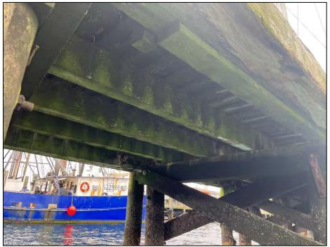
Photo No. 12.: View of the typical weathered stringer and decking condition below the timber pier south of the building pier.
