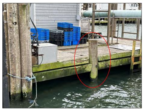
Photo No. 8.: Damage due to impact on the west face of the pier.
