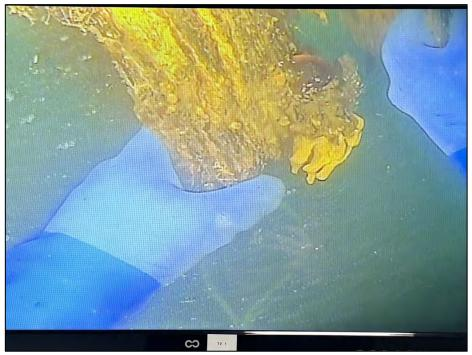
Photo No. 9.: View of the disconnected pile condition near the mudline of the pile in photo 8.
