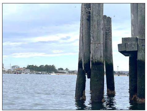
Photo No. 6.: Damaged condition of the eastern dolphin pile at the head of the pier.
