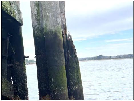
Photo No. 5.: Damaged condition of the western dolphin pile at the head of the pier.
