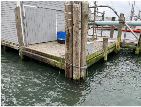
Photo No. 7.: View of the timber pier at the head of the building pier. The timber pier is a separate foundation system than the building pier.
