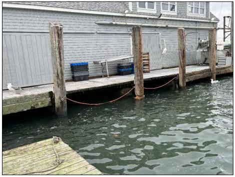
Photo No. 10.: Missing exterior stinger and chocks on the south face of the timber Pier I between bent 2 and bent 4.
