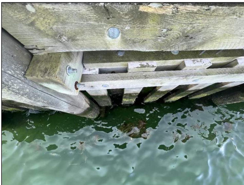
Photo 6. Existing wave boards viewed from above
