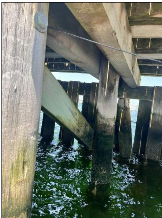
Photo 9. Typical framing of fixed piers, battered piles face the northwesterly direction
