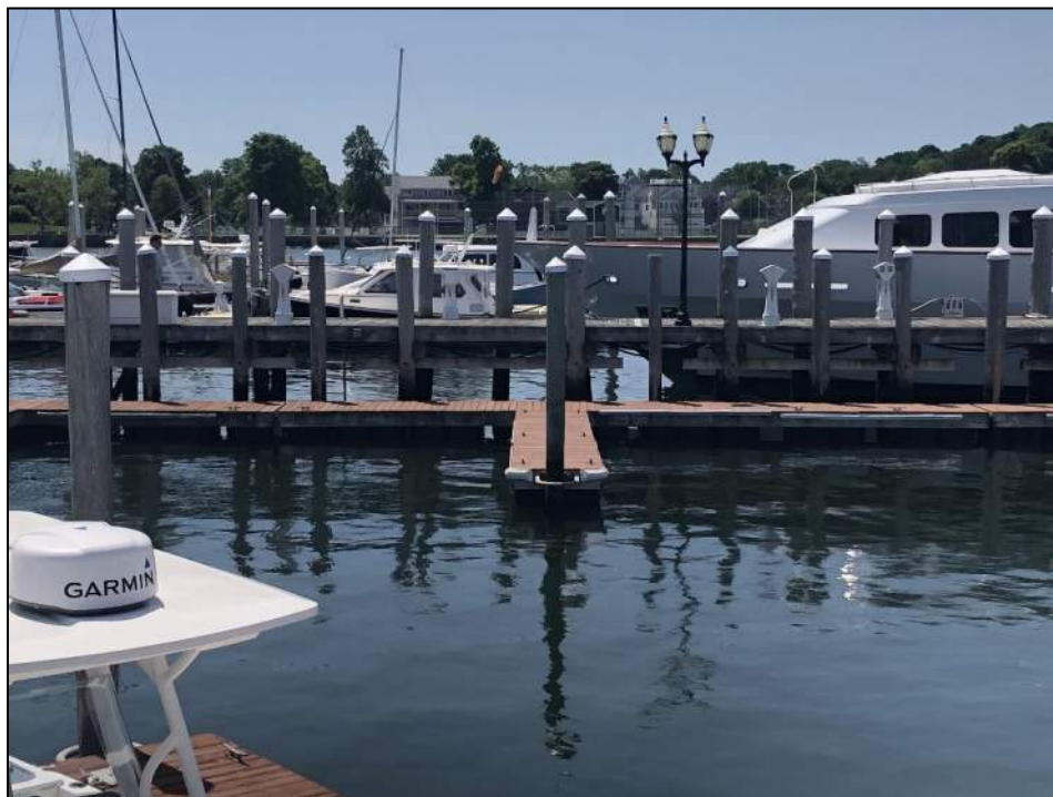
Photo 11. Spacing of existing pier piles, no wave boards along protected southern side.
