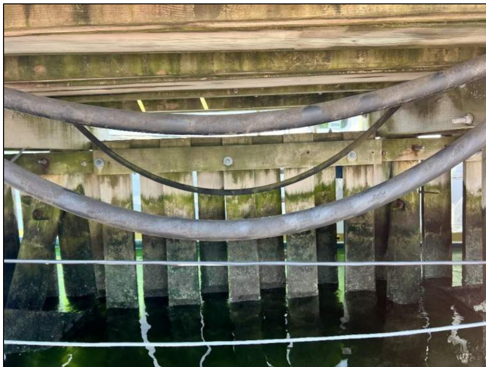
Photo 7. Existing wave boards viewed from back
