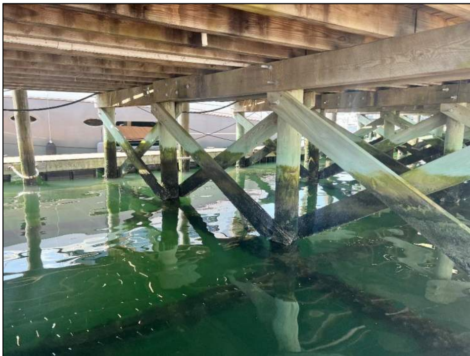
Photo 3. Typical framing under existing deck (to remain)
