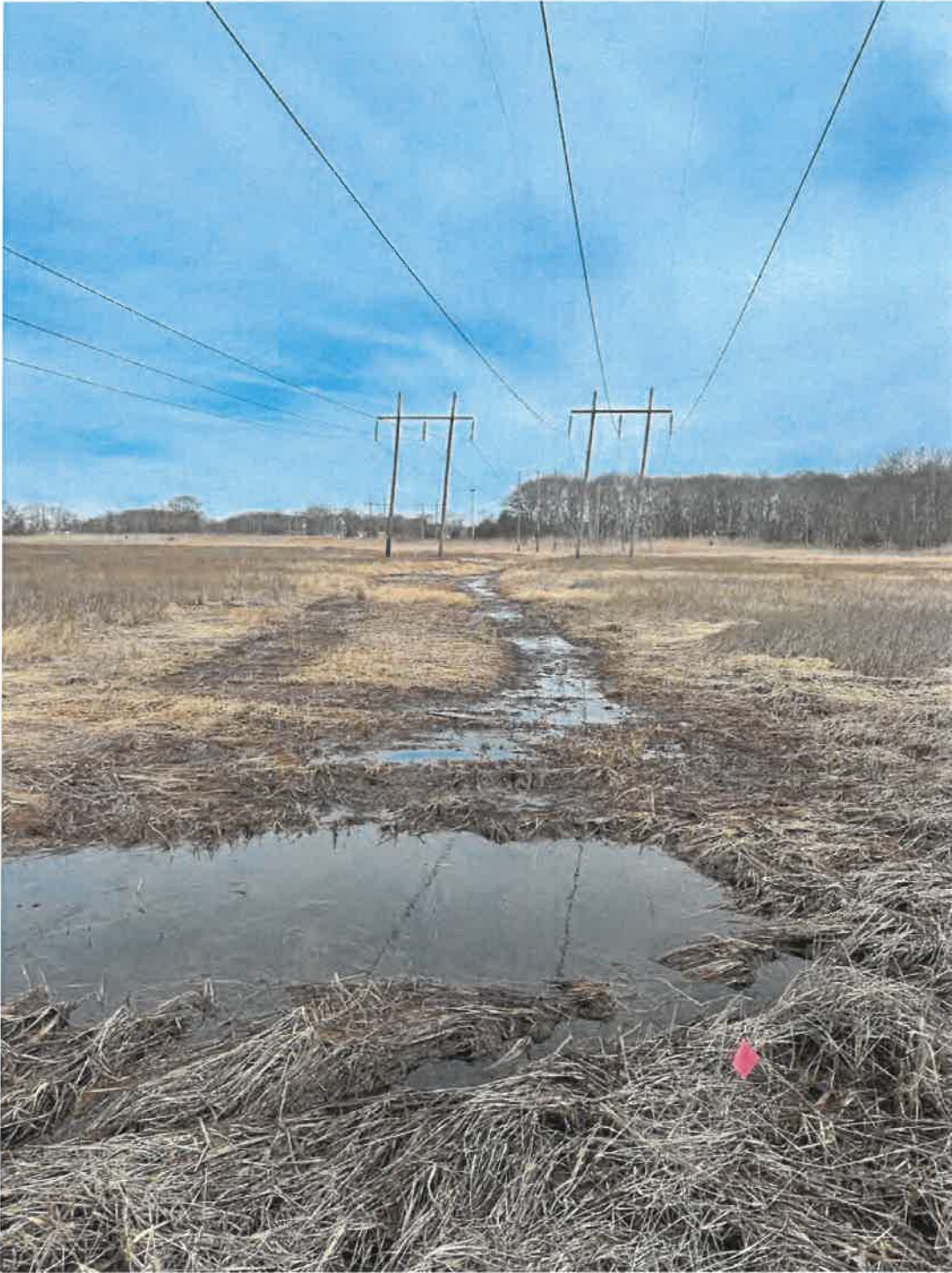
(Figure 1: Standing water in areas of compacted peat along vehicles tracks from work performed in January 2025. Picture taken March 18, 2025)
