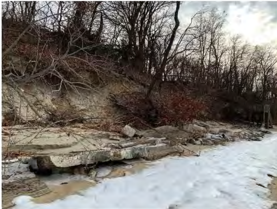
Photo 6: Significant erosion of slope, downed trees on beach and unstable trees on slope from December 23, 2022 storm.
