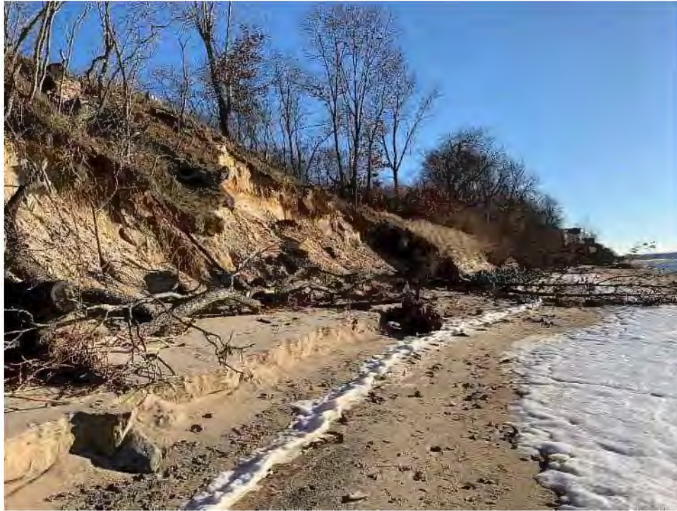
Photo 1: Overview of shoreline looking south. Note significant erosion and downed trees from December 23, 2022 storm
