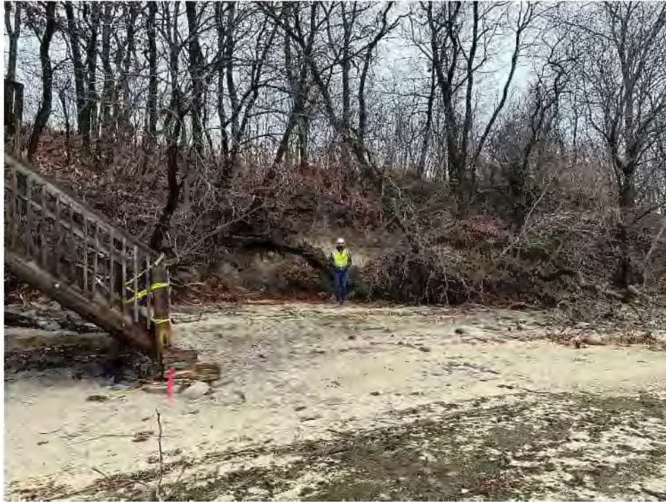
Photo 9: Significant erosion of slope, damaged stairs, downed trees on beach and unstable trees on slope from December 23, 2022 storm. The individual in the photo is 6'-3" for reference.
