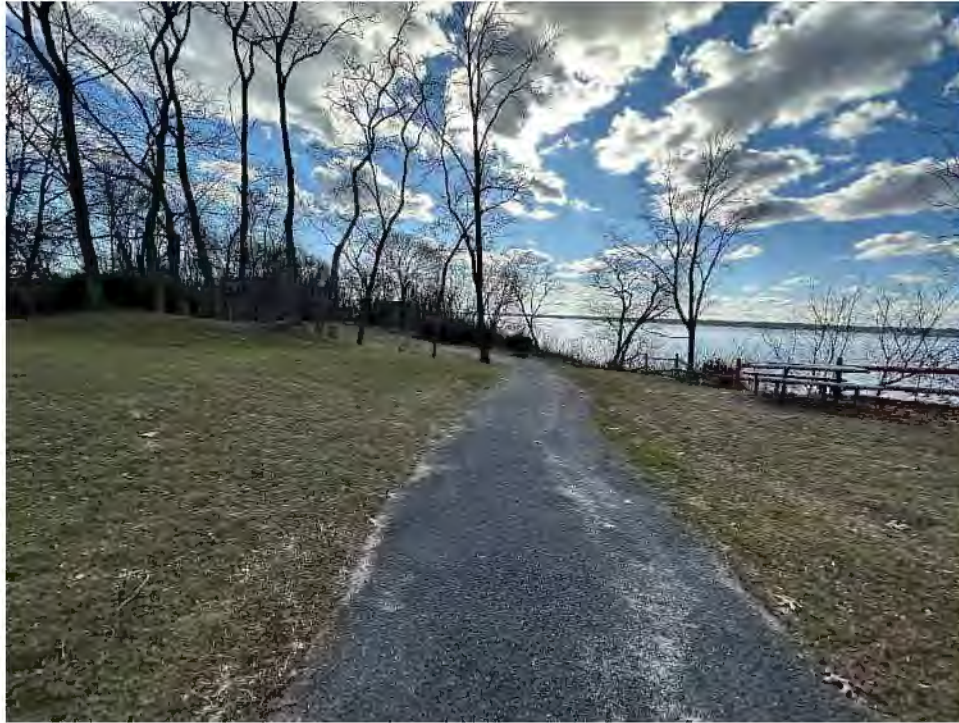
Photo 13: Overview of area behind slope at northern end of work, looking south.
