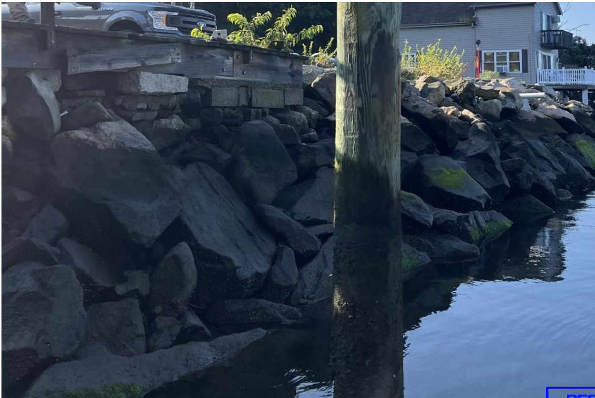
Photo No.6: View of existing riprap slope and timber pad adjacent to parking area.
