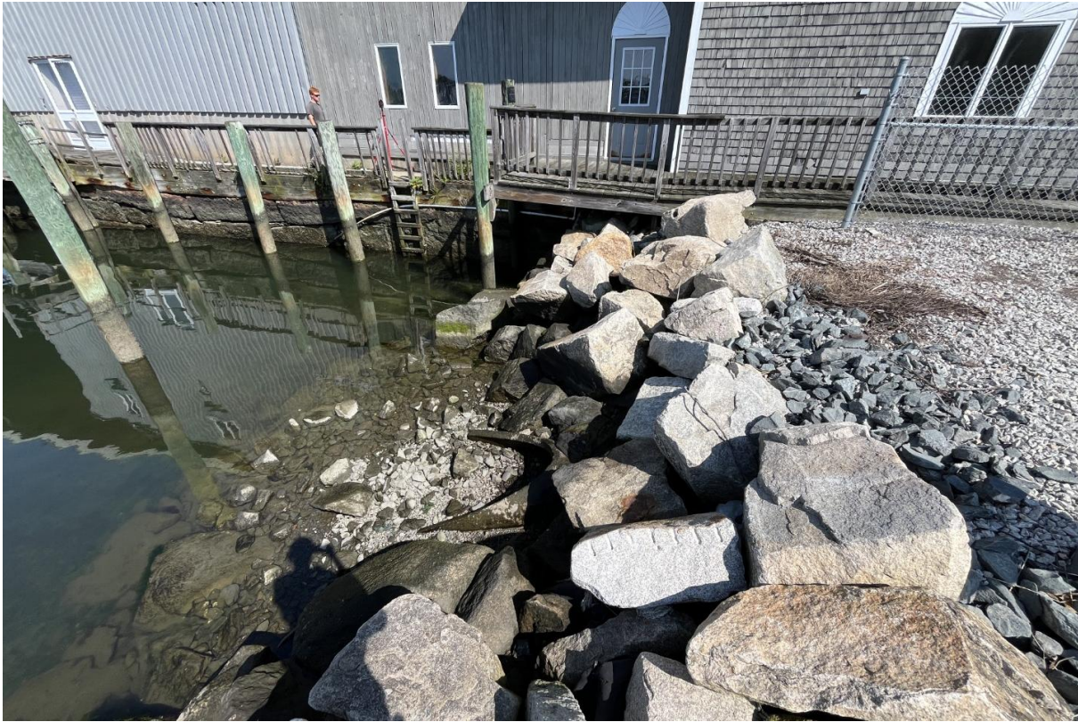
Photo No.7: View of existing riprap slope, parking area, and timber walkway along the building.
