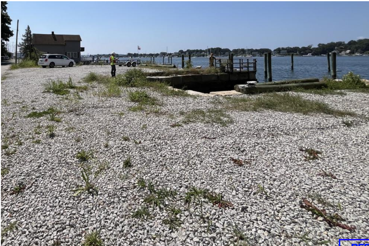
Photo No.8: View looking south, of existing parking area with previous railroad basin.
