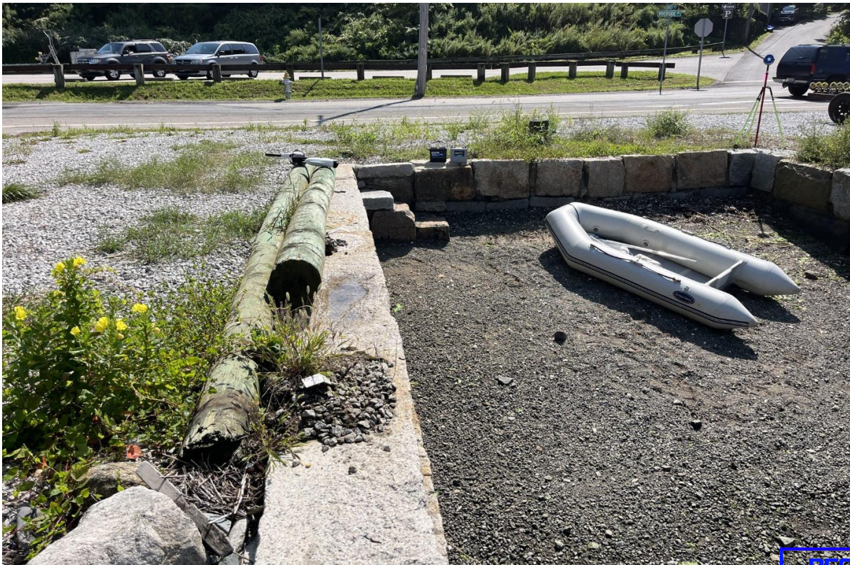
Photo No.2: Previously decommissioned marine railway basin to be filled.
