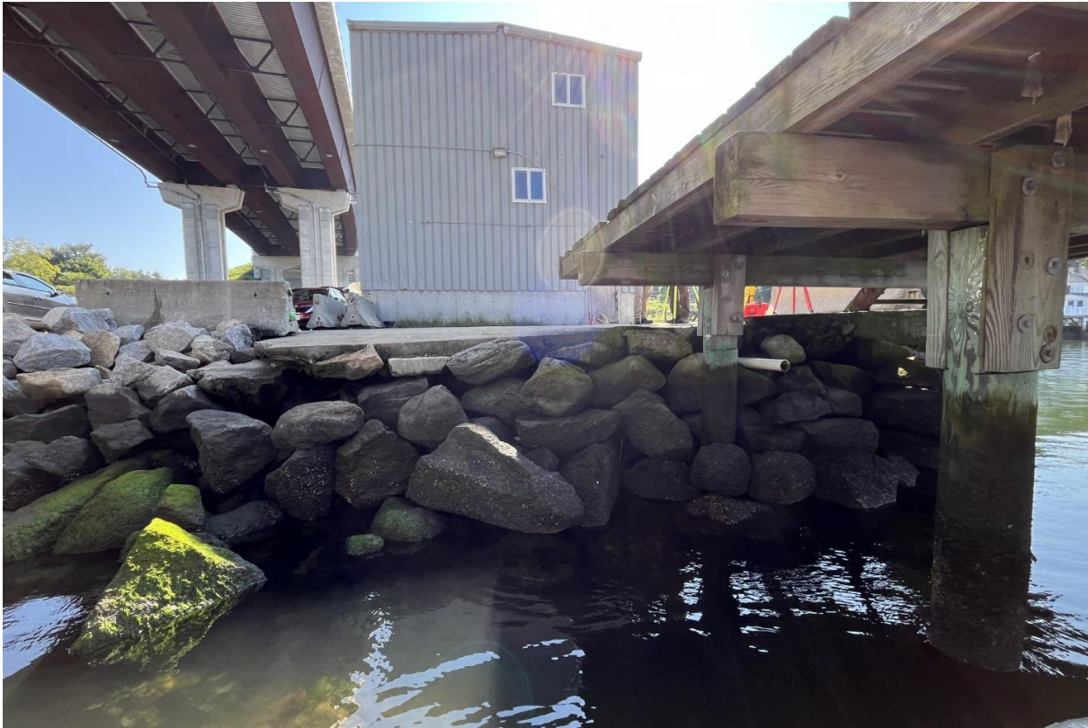
Photo No.5: View of existing timber pier and concrete pad to be replaced.
