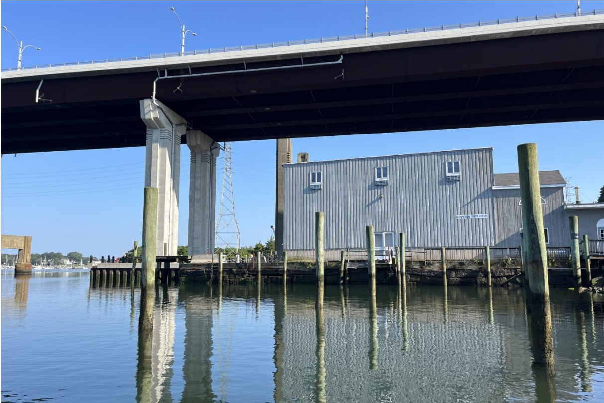
Photo No.1: View looking north of existing building, timber pier, and pilings.
