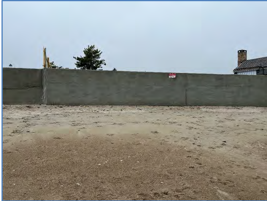
Figure 3: Western Section of Seawall at Property Line
