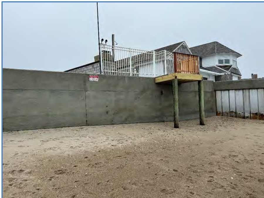
Figure 4: Western Section of Seawall and Access Stairs
