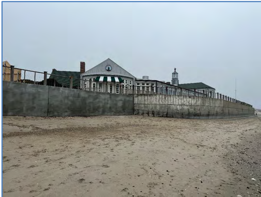
Figure 16: Concrete Seawalls Facing Northeast at Property Line
