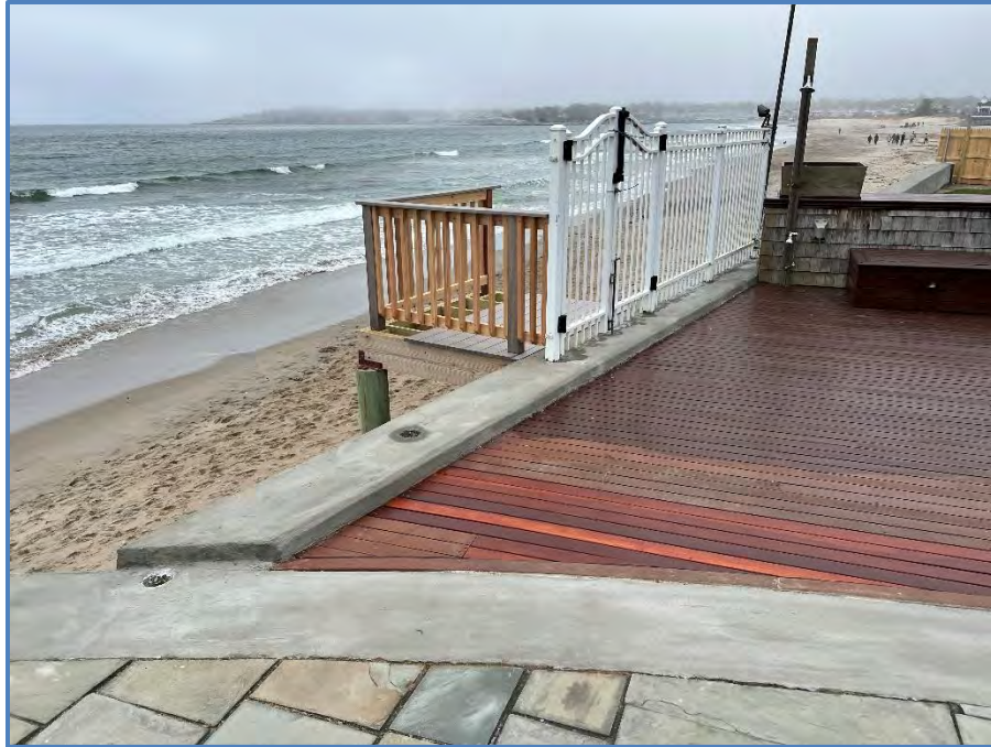
Figure 9: Upland behind Western Section of Seawall near Access Stairs
