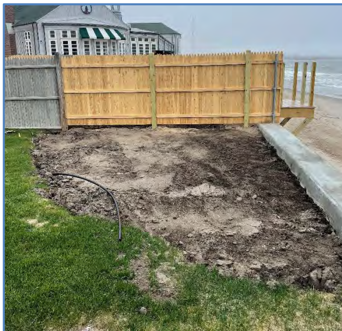
Figure 13: Area Restored From Undermining
