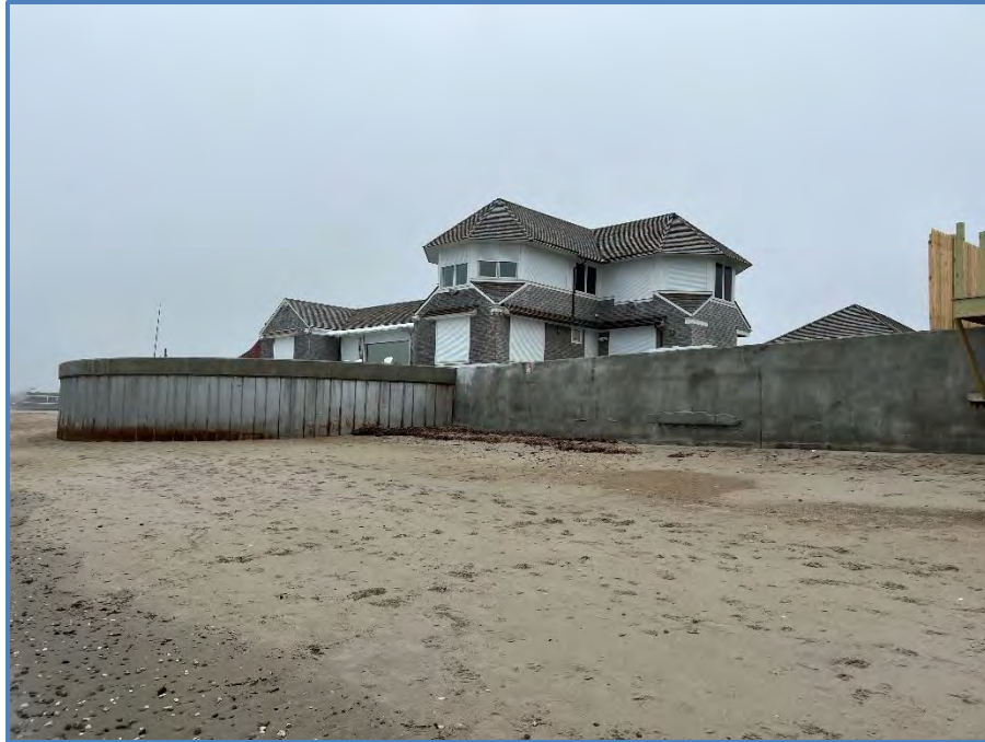
Figure 7: Middle Section with Curved Bulkhead and Eastern Side of Seawall
