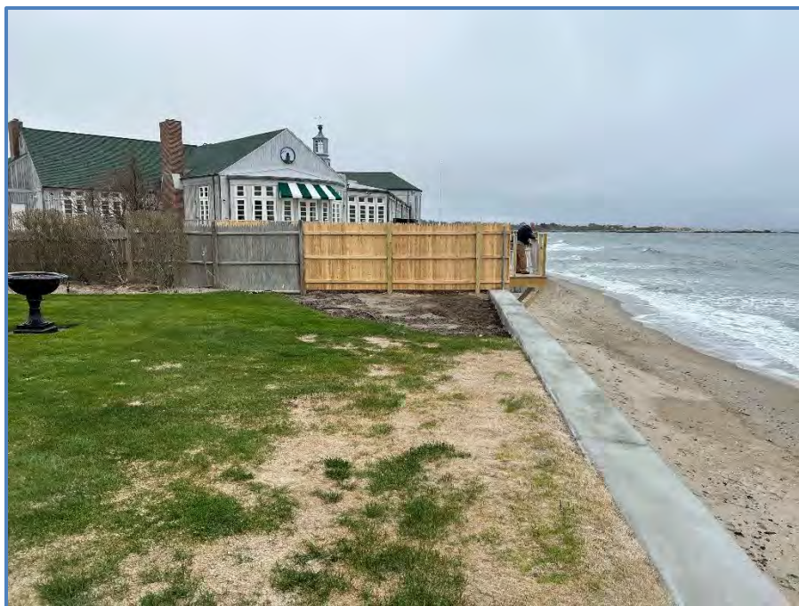
Figure 11: Upland behind Eastern Section of Seawall
