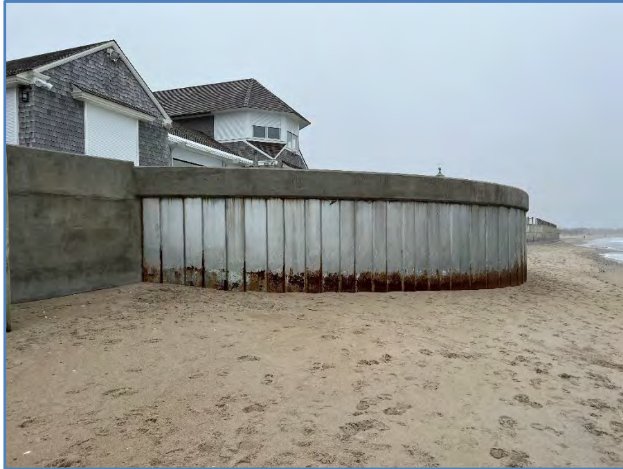
Figure 5: Middle Section with Curved Bulkhead
