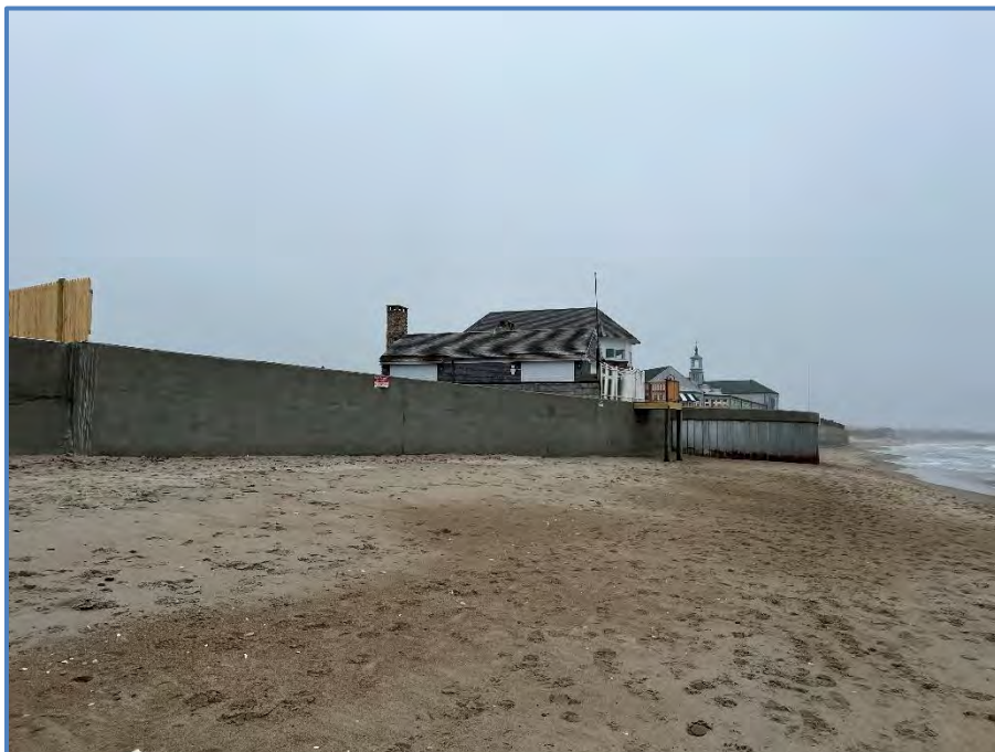
Figure 2: Western Section of Concrete Seawall and Steel Bulkhead
