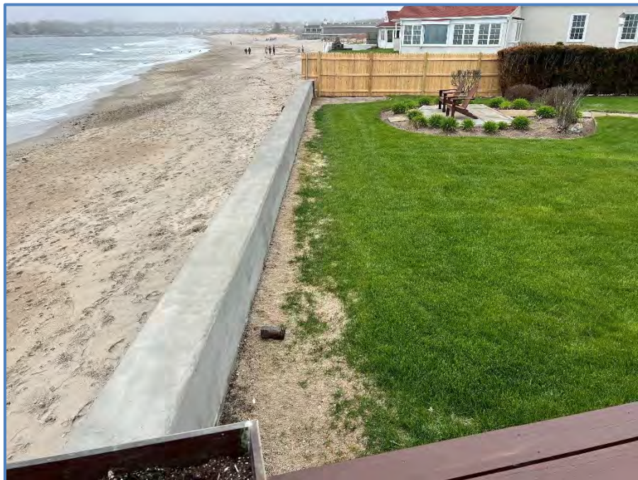
Figure 8: Upland behind Western Section of Seawall
