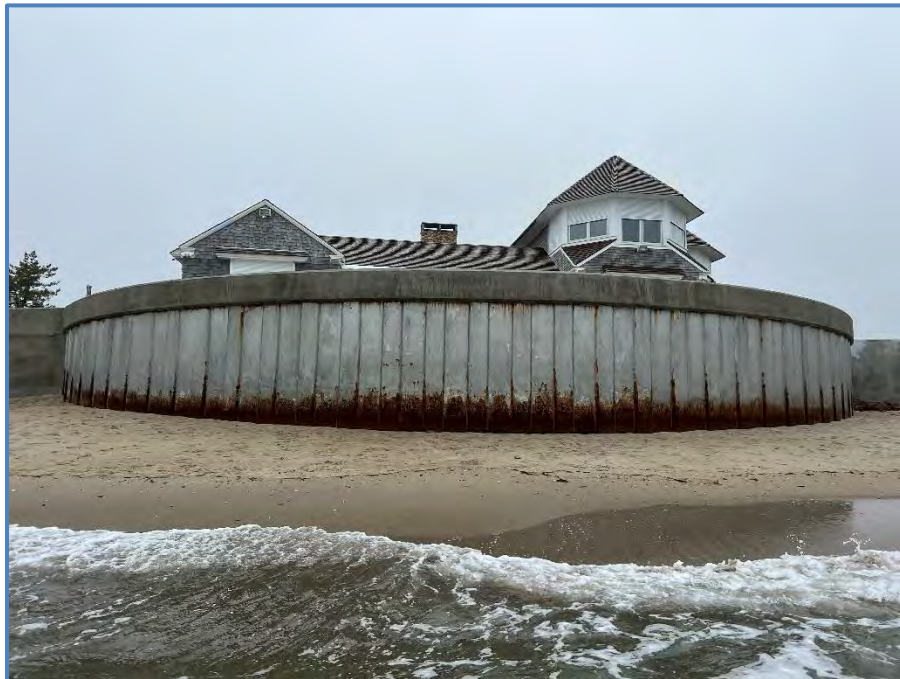
Figure 6: Middle Section with Curved Bulkhead
