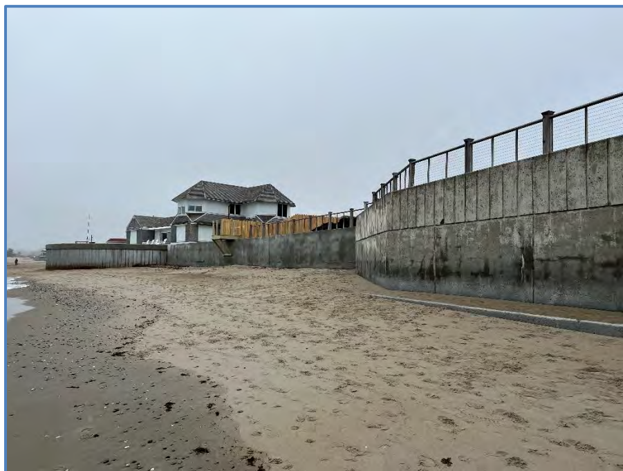
Figure 3: Concrete Seawalls Facing Northwest
