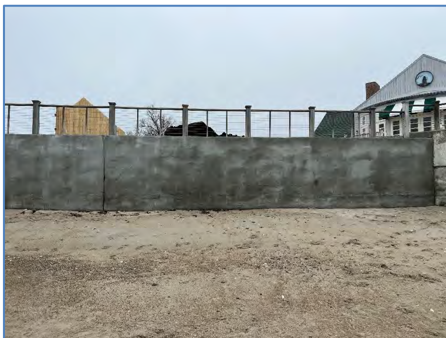
Figure 4: Older Section of Concrete Seawall
