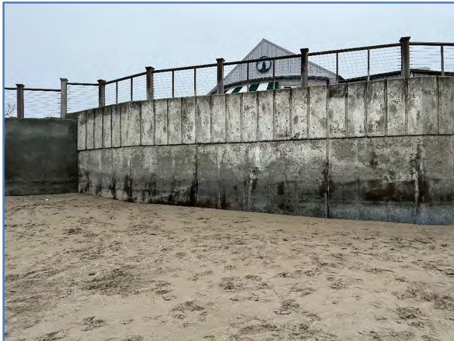
Figure 5: Start of Newer Section of Concrete Seawall
