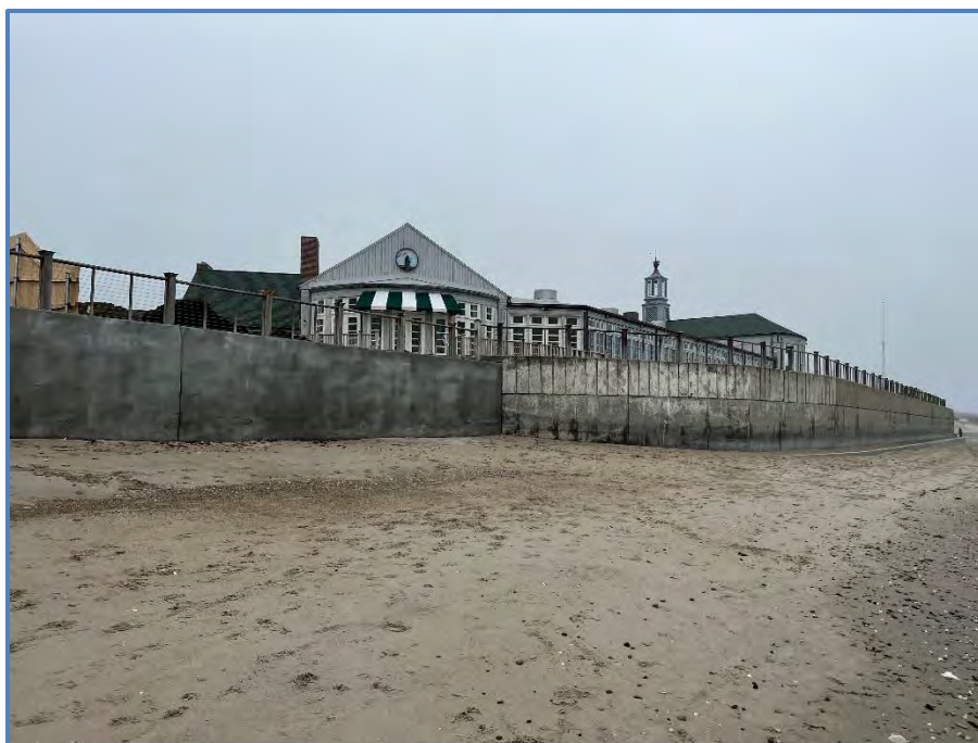
Figure 2: Concrete Seawalls Facing Northeast
