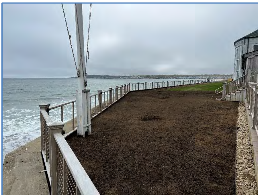
Figure 10: Upland near Return Section of Seawall
