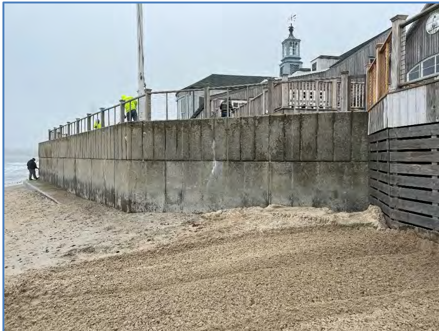
Figure 9: Return Section of Seawall
