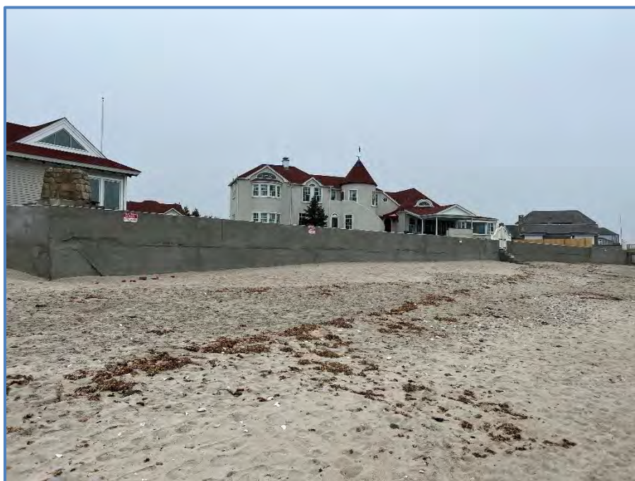
Figure 4: Seawall facing Northeast
