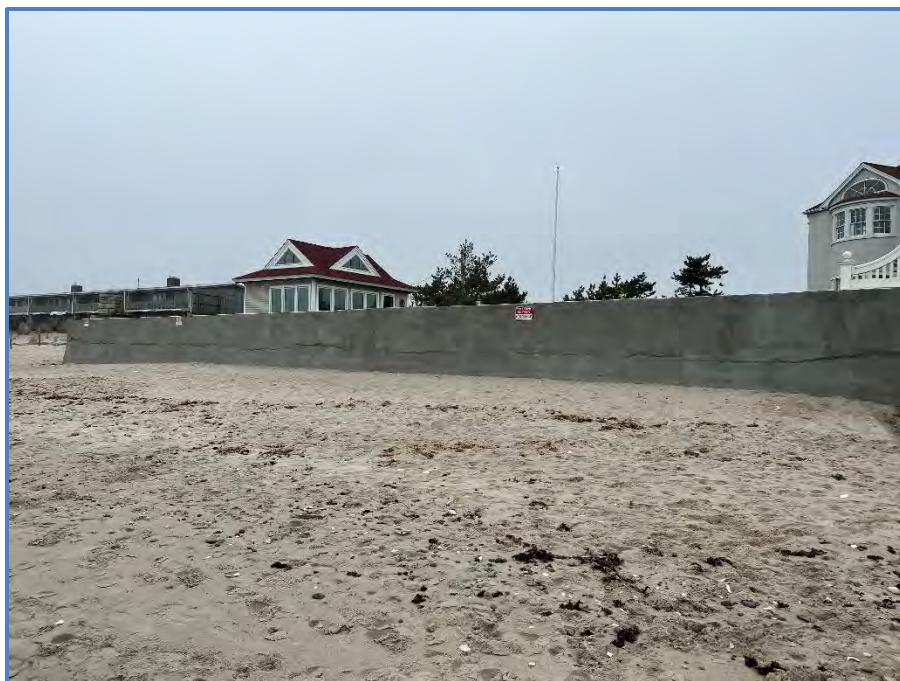
Figure 5: Western Side of Seawall
