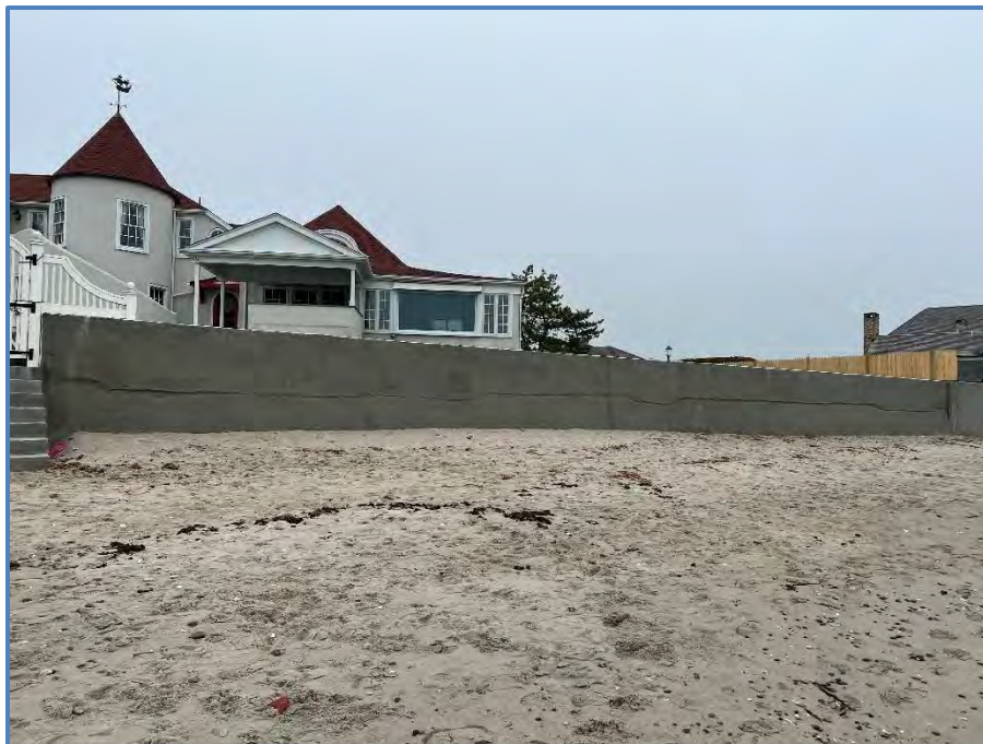
Figure 7: Eastern Side of Seawall
