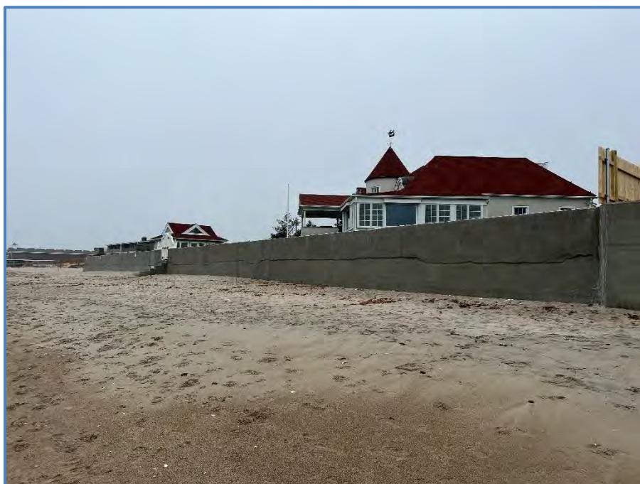
Figure 8: Seawall facing Southwest
