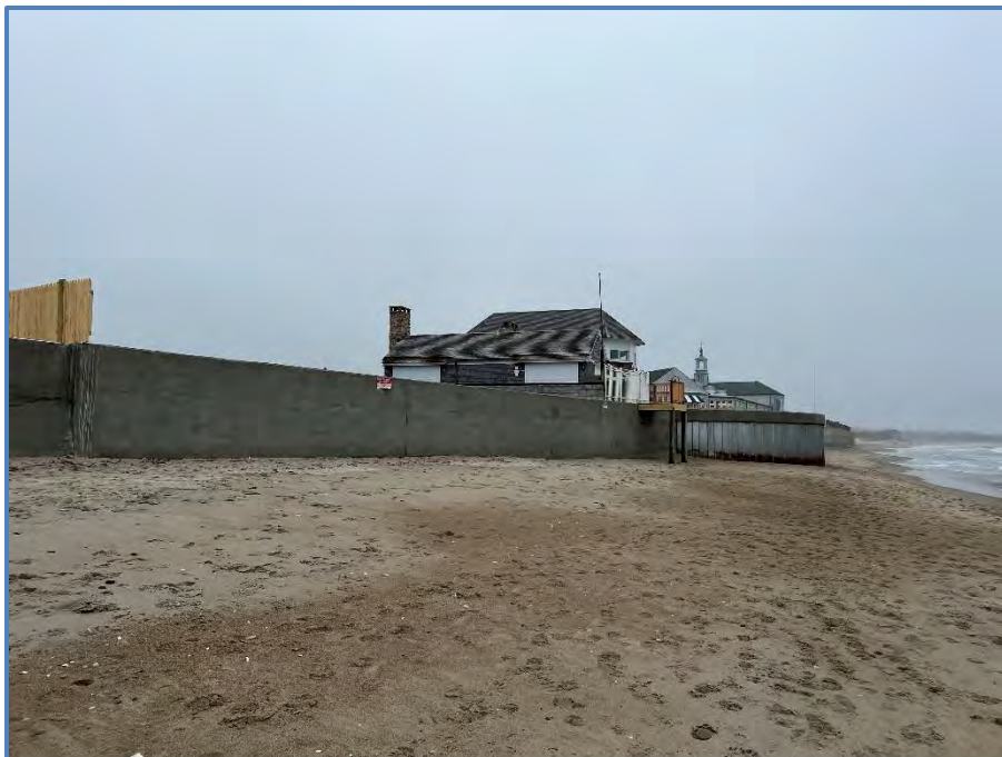
Figure 11: Section of Concrete Seawall and Steel Bulkhead at Eastern Property Line
