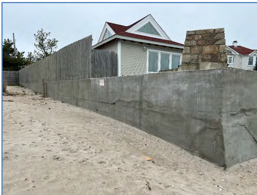
Figure 3: Concrete Return Wall
