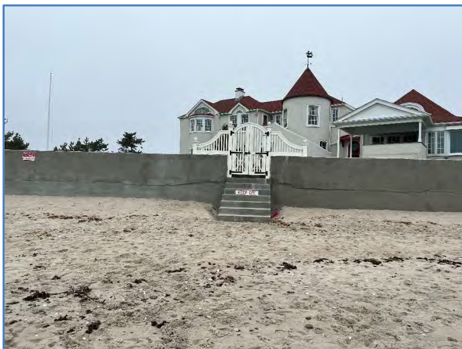
Figure 6: Center of Seawall at Stairs
