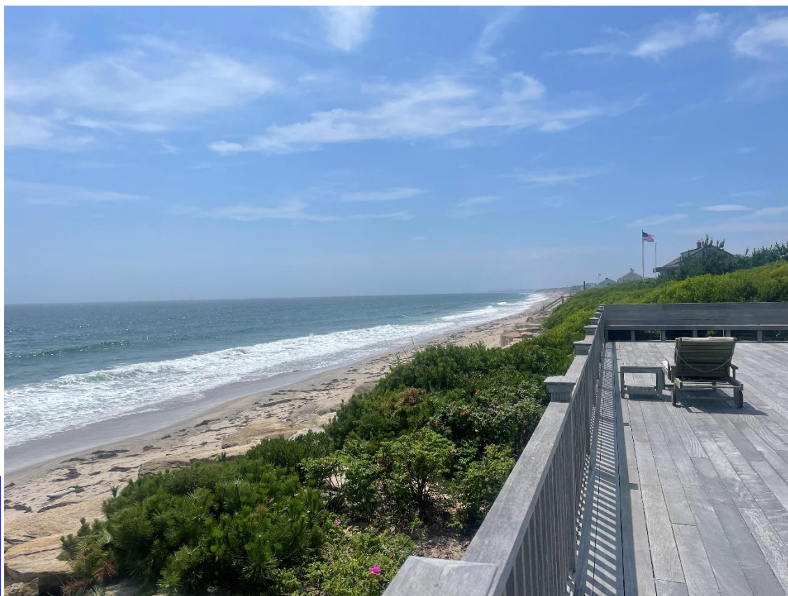
Photo 2: Existing top of revetment and buffer (looking west).
