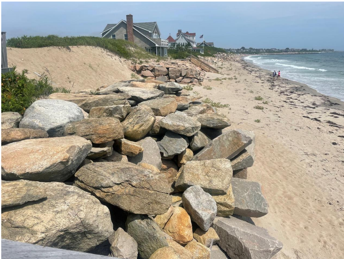
Photo 4: Existing revetment; taken from existing stairs looking east.
