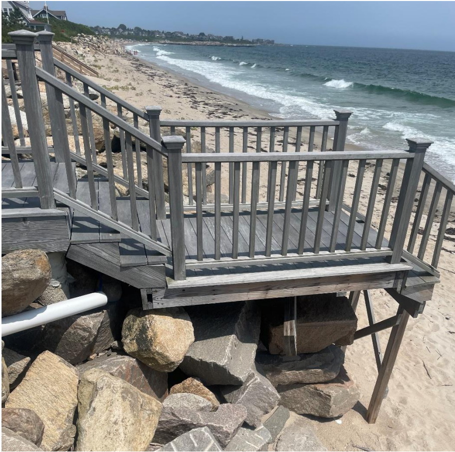
Photo 5: Existing stairs looking west.
