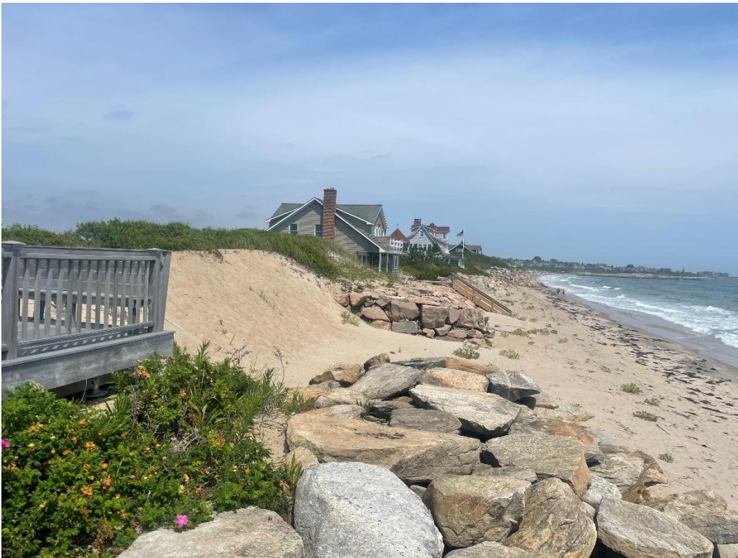
Photo 6: Existing area of proposed infill structural shoreline protection.
