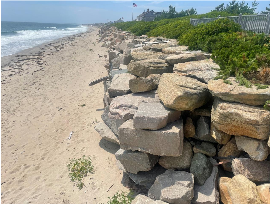
Photo 3: Existing revetment; taken from existing stairs looking west.
