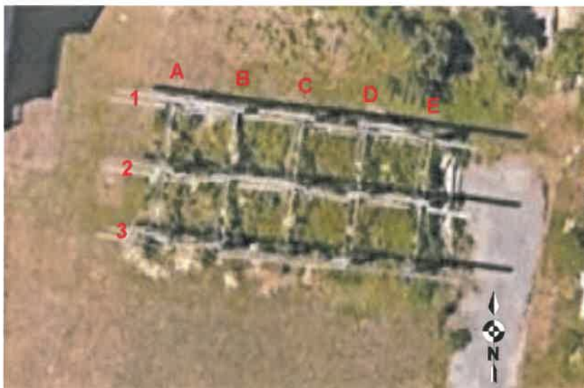
Figure 2. Google Maps Imagery of Project Location
