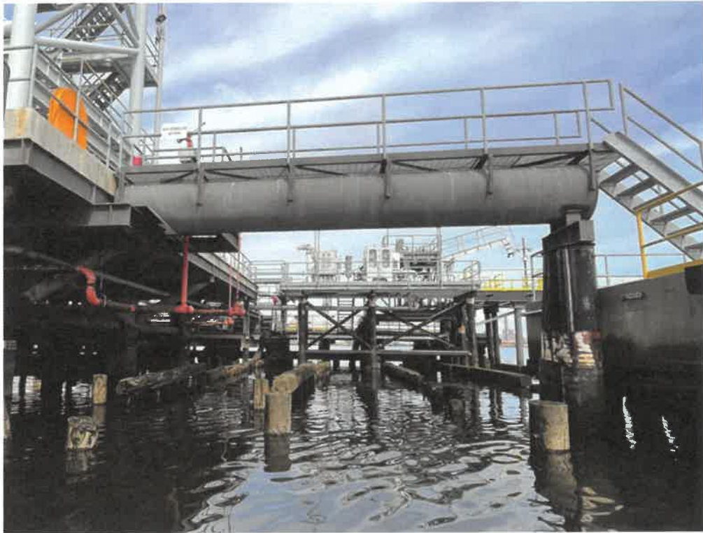
Photo 10: Southern steel catwalk.
