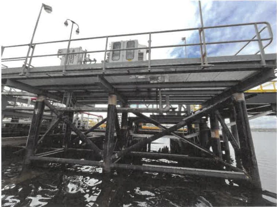
Photo 14: Barge gangway platform.
