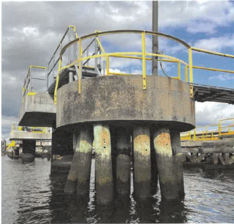
Photo 1: Northern abandoned timber supported concrete mooring dolphin.
