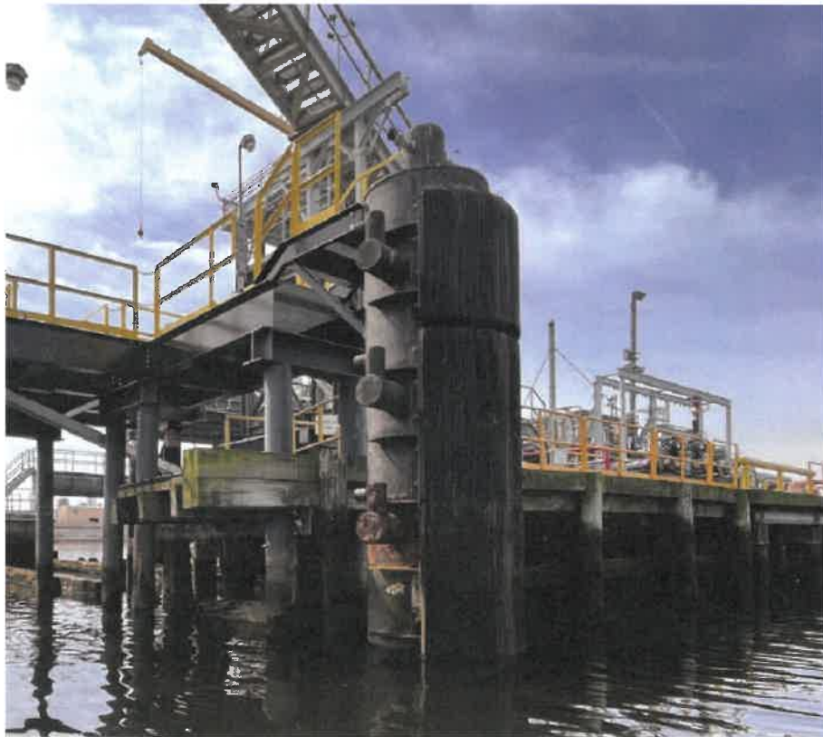
Photo 3: Steel monopile breasting dolphin M3. (Typical configuration for M1, M2, M3 & M4)
