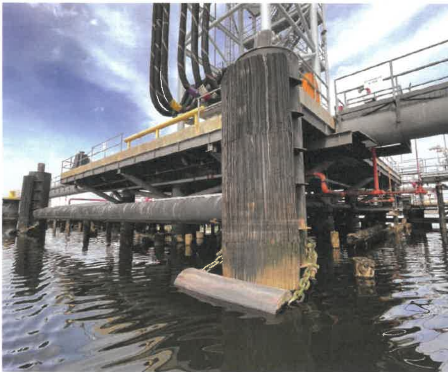
Photo 8: Steel monopile breasting dolphin M5. (Typical configuration for M5 & M6)
