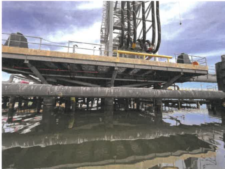
Photo 12: Hose tower platform.
