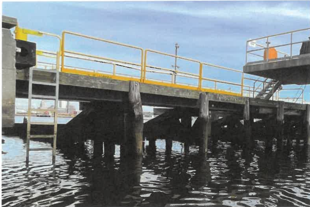
Photo 9: Southern timber catwalk.
