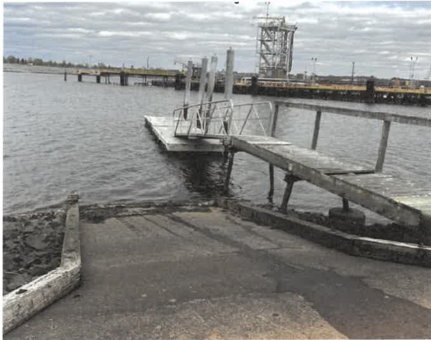
Photo 17: Boat ramp and floating dock.
