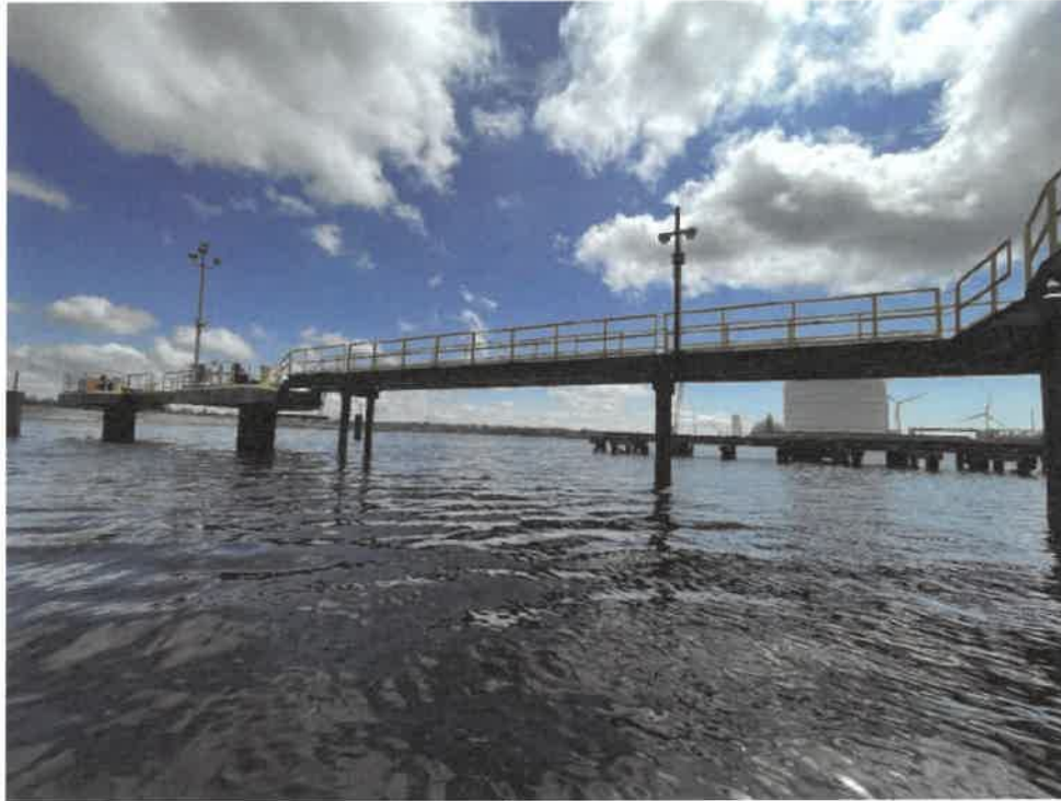
Photo 5: Northern steel catwalk.
