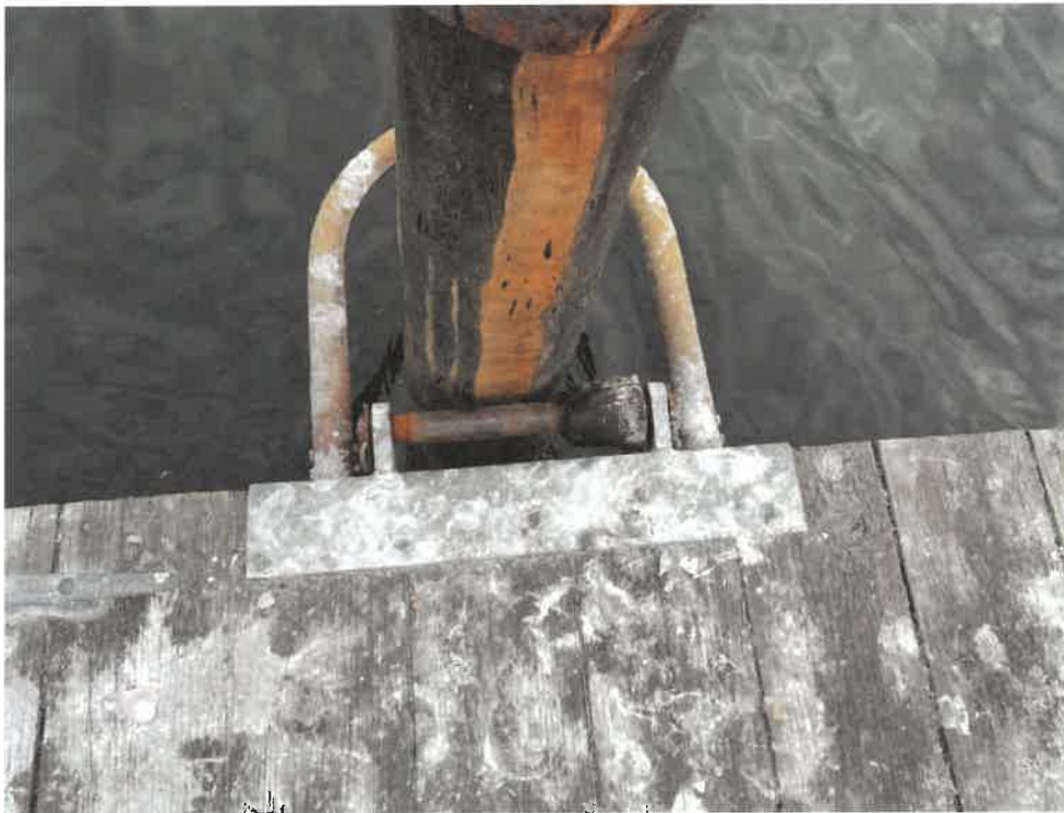
Photo 18: Boat ramp and floating dock pile guide.
