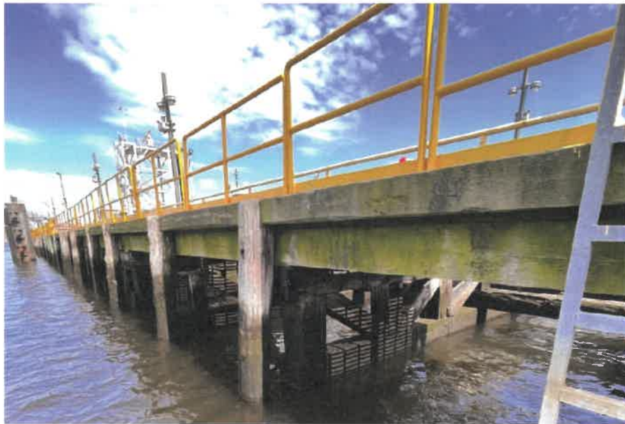
Photo 4: Northern timber catwalk.
