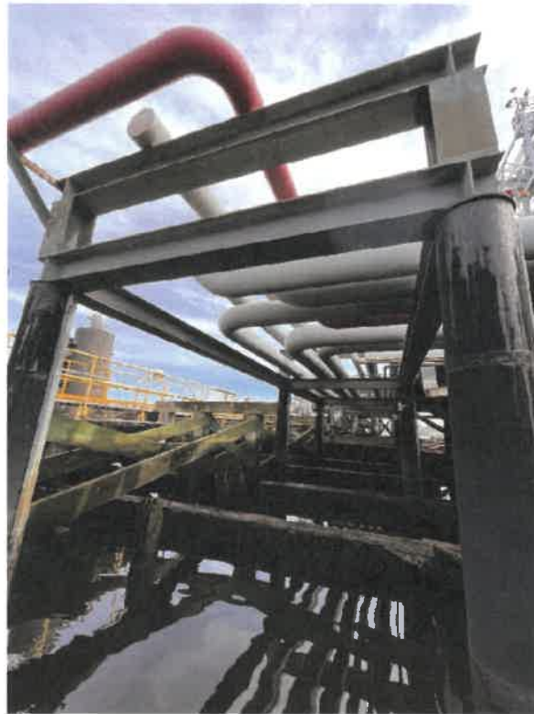
Photo 16: Northern steel pipe rack.
