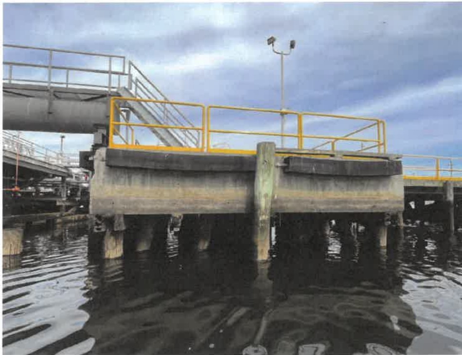
Photo 6: Southern abandoned timber supported concrete mooring dolphin.
