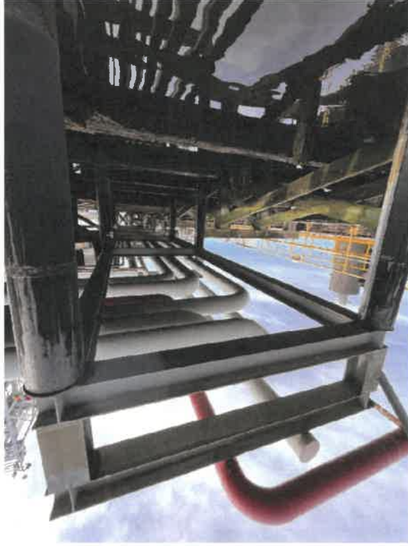
Photo 16: Northern steel pipe rack.
