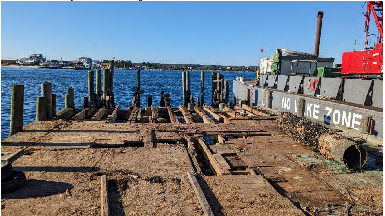
View of structurally deficient framing.
