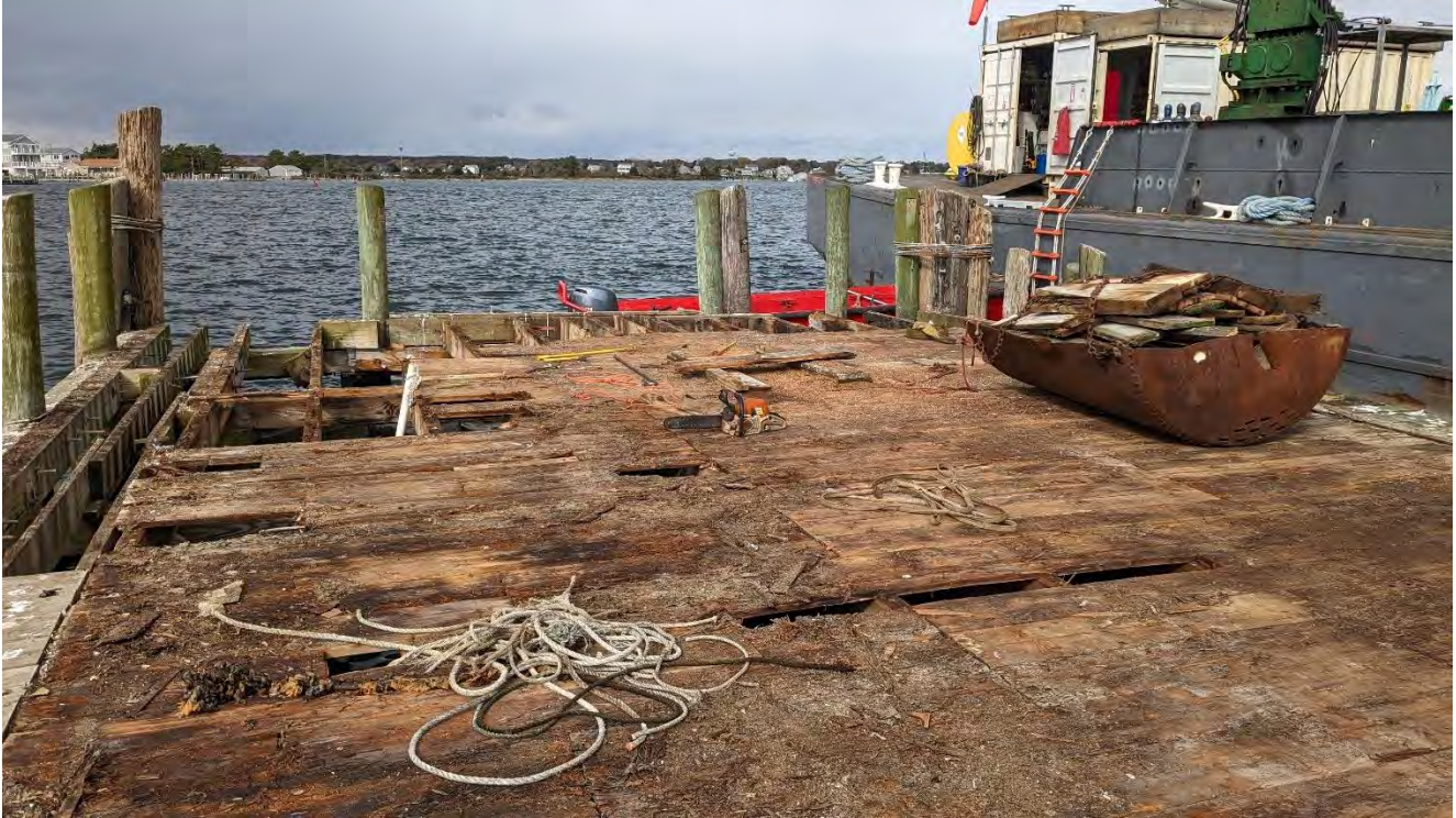
After Removal of the Plywood surface holding the dock together
