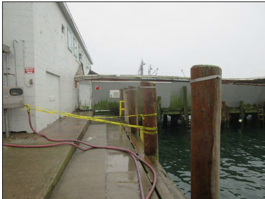
Photo 4: Original pier elevation continuing at an elevation higher than the existing bulkhead to connect to the landside buildings FFE.
