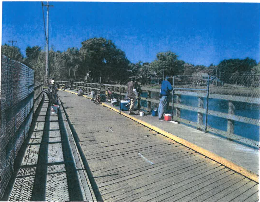
Fishing off the Warren/Palmer River span, clearly showing “sidewalks” (Photo: www.trailink.com )
