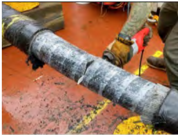
Figure 6. Representative Out-of-service Cable Cutting Operation on PLGR Vessel
