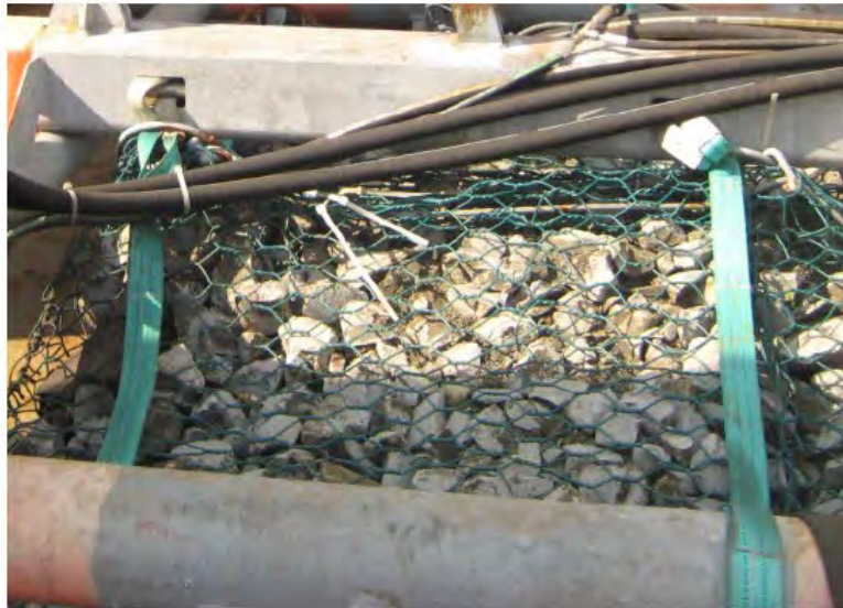
Figure 16. Rock Gabion in Concrete Mattress Handling Frame
