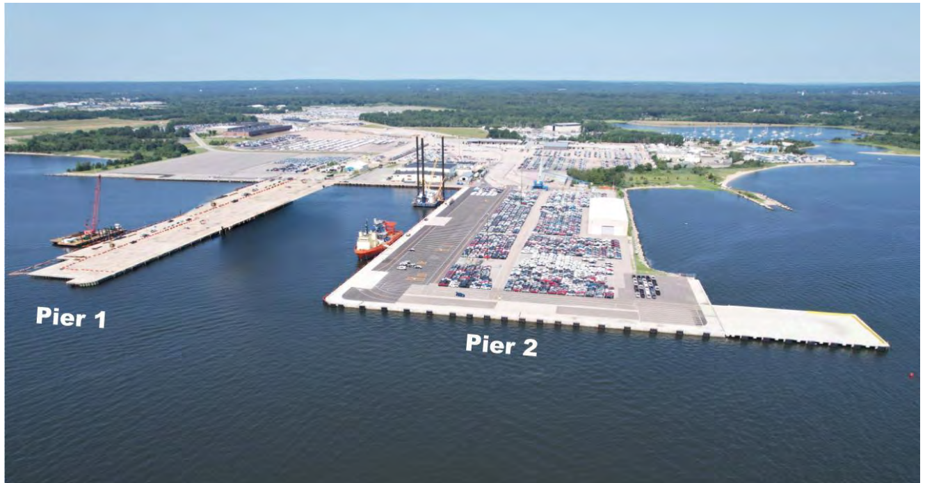
Photo 1: Port of Davisville's Pier 1 and Pier 2 facing west.
