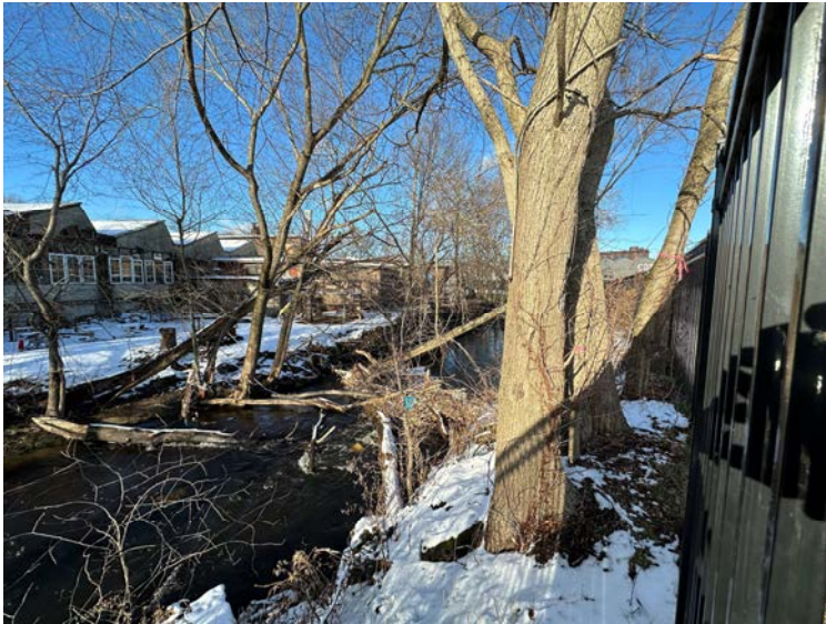
FIGURE 1L – RECENT FLOOD EVENTS CREATED A SEDIMENT AND TRASH DAM AT THE SITE OF THE RECENTLY CONSTRUCTED GOTHAM GREENS BIKE PATH.
