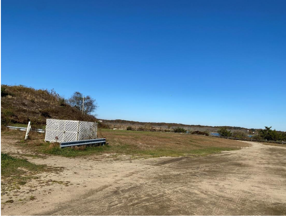
#5 View of area to the Rear of the Building facing Northerly
