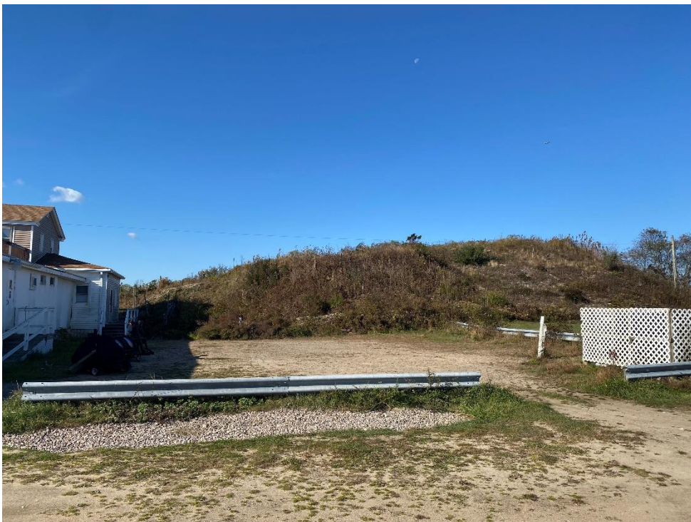
#4 View of Rear of Building facing Westerly
