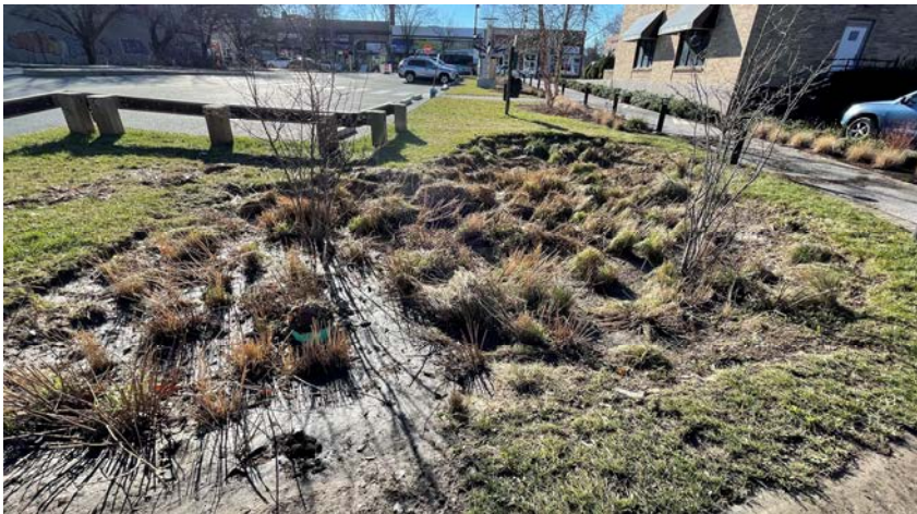
FIGURE 1C – BIORETENTION BASINS INSTALLED JUST SOUTH OF SAN SOUCI DRIVE. FLOODING FROM THE RIVER AFTER DECEMBER 18, 2023 RAINFALL EVENT HAS FILLED THE BASINS WITH SILT AND MUD.
