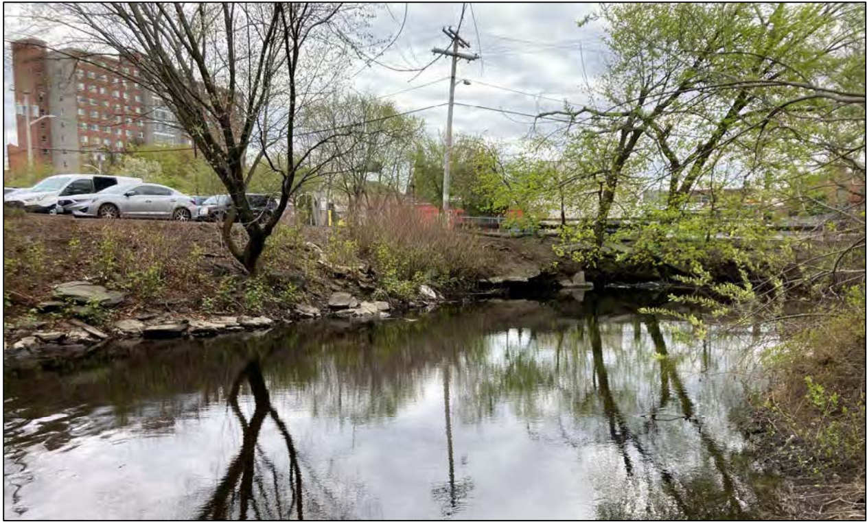
Photo 1: Undercut bank across the Woonasquatucket River, looking south (19 April 2023)
