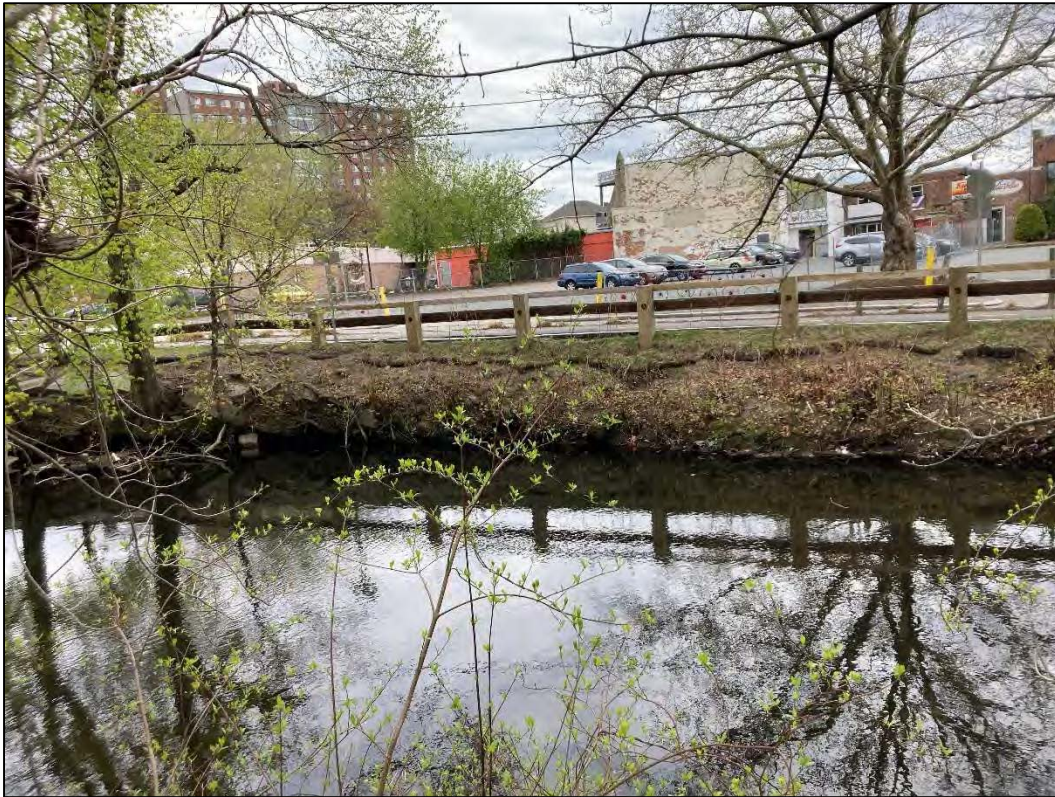
Photo 3: Upstream end of undercut bank on river right, looking south (19 April 2023)
