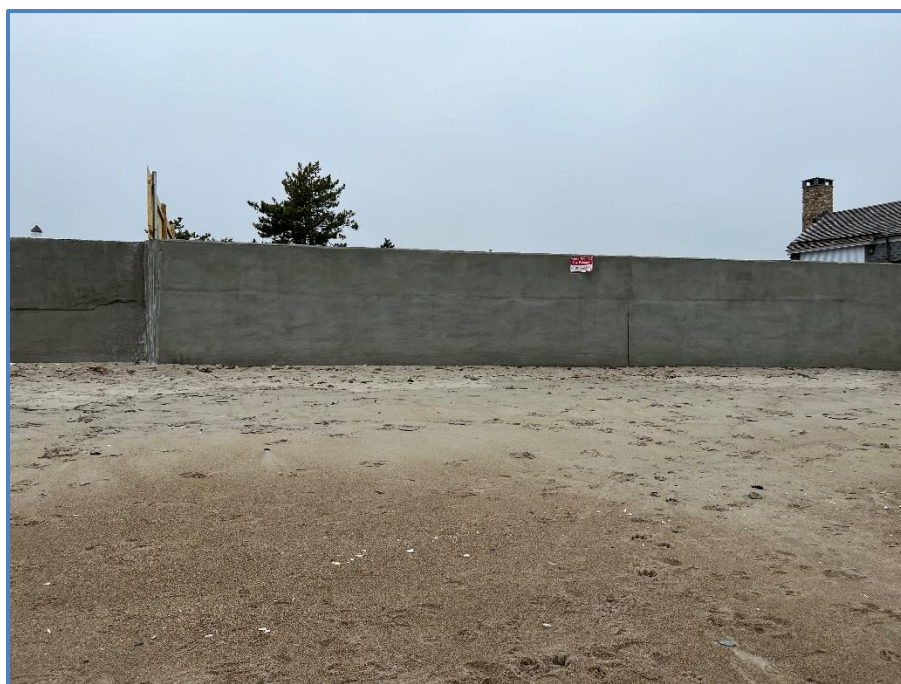
Figure 12: Western Section of Seawall
