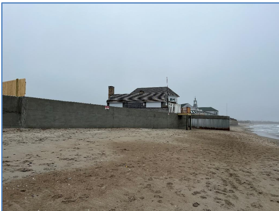
Figure 11: Western Section of Concrete Seawall and Steel Bulkhead
