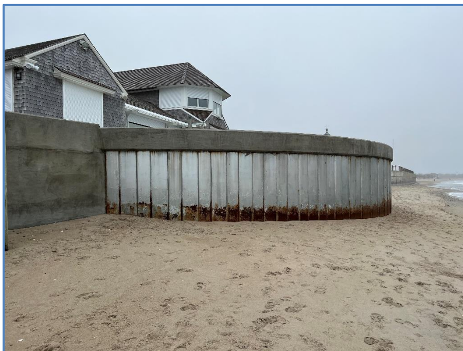
Figure 14: Middle Section with Curved Bulkhead
