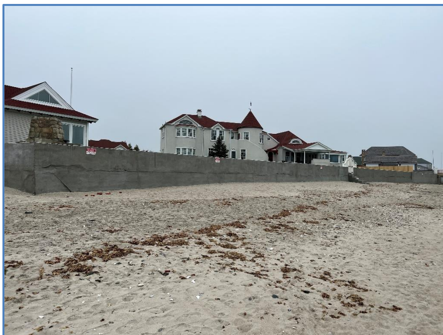
Figure 4: Seawall facing Northeast
