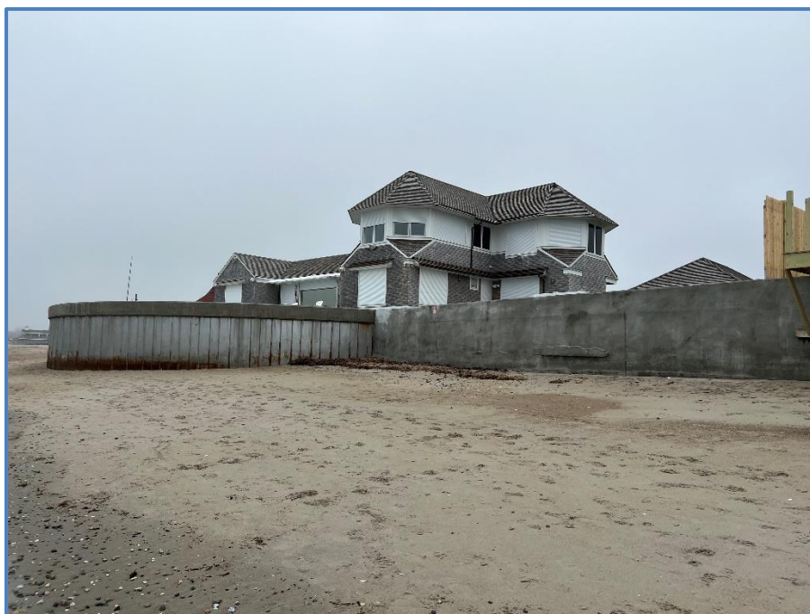
Figure 16: Middle Section with Curved Bulkhead and Eastern Side of Seawall
