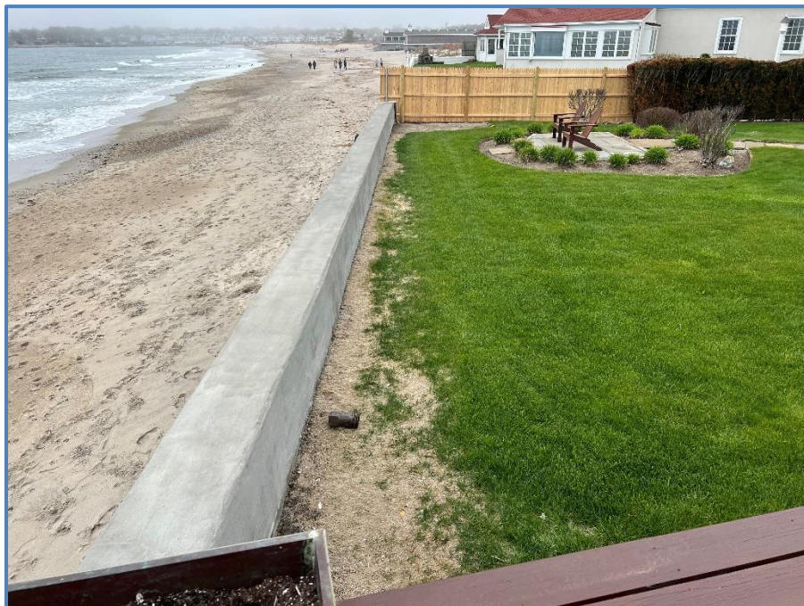
Figure 17: Upland behind Western Section of Seawall
