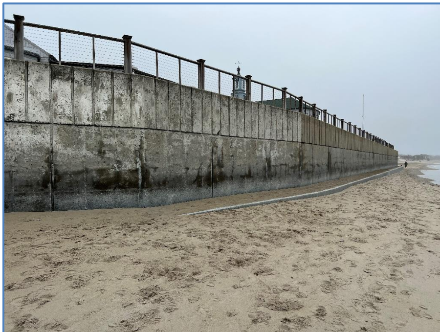
Figure 29: Concrete Seawall Facing Northeast
