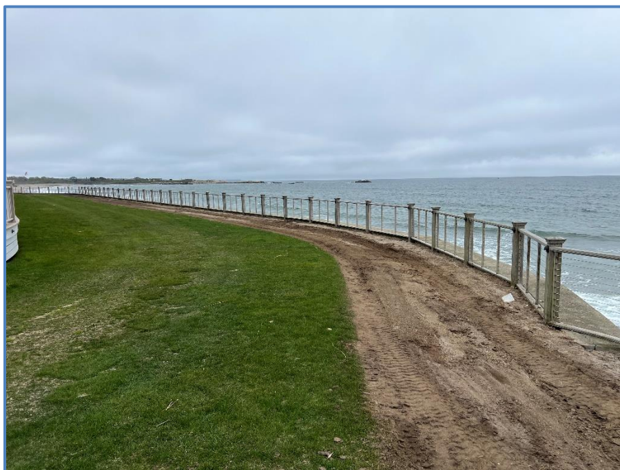
Figure 36: Upland Area Along Seawall
