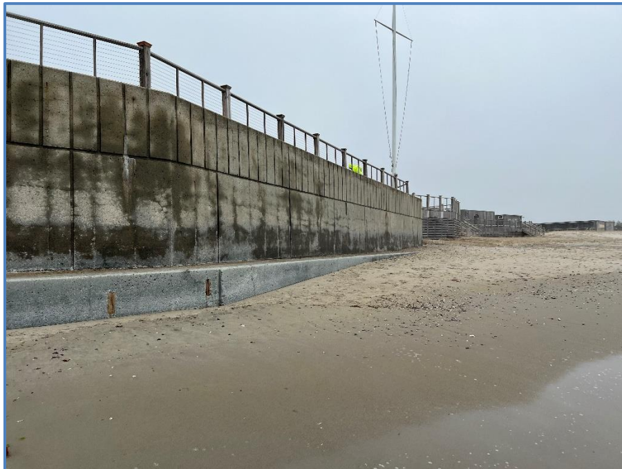
Figure 31: Start of Return Section of Seawall
