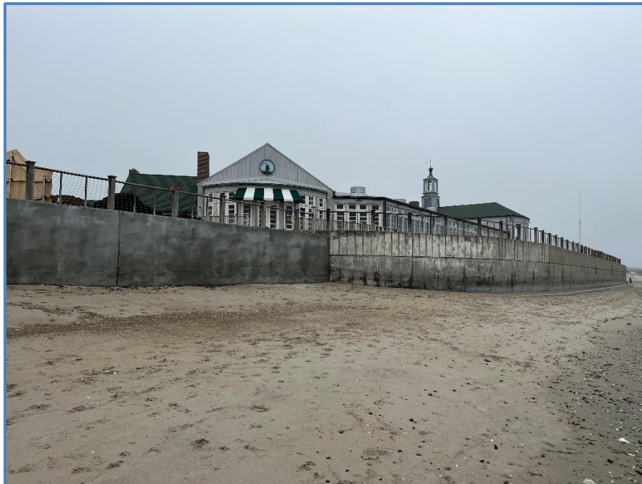
Figure 25: Concrete Seawalls Facing Northeast
