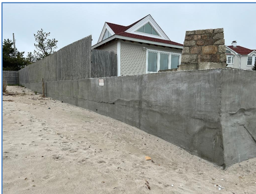
Figure 3: Concrete Return Wall
