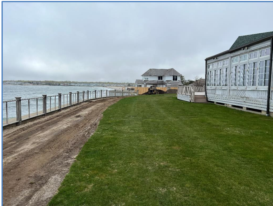
Figure 35: Upland Area Along Seawall
