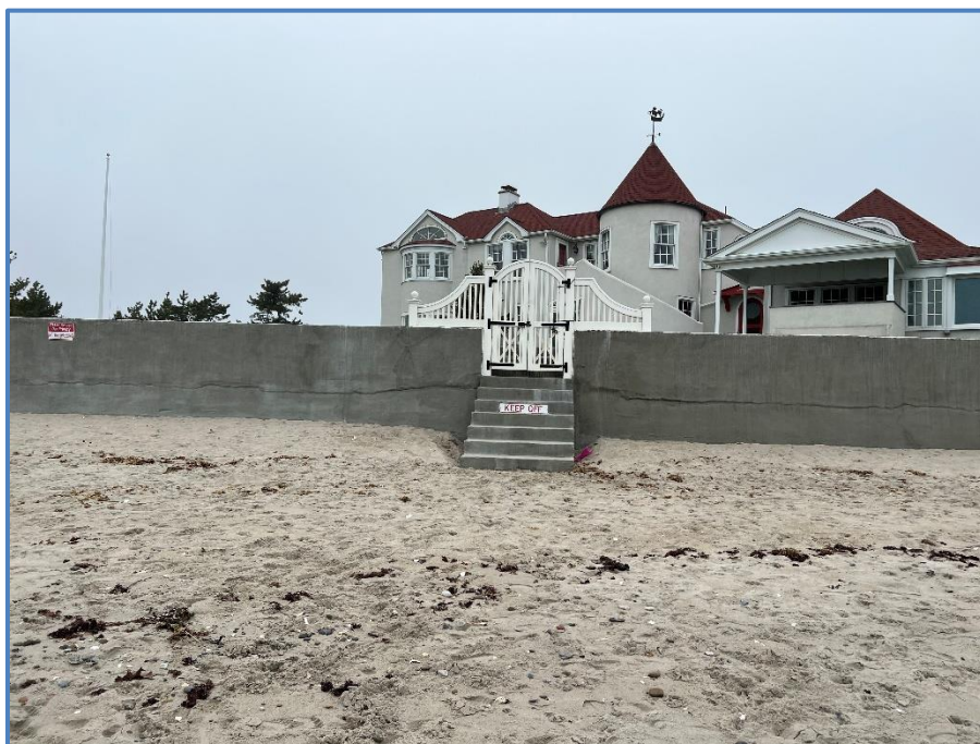
Figure 6: Center of Seawall at Stairs
