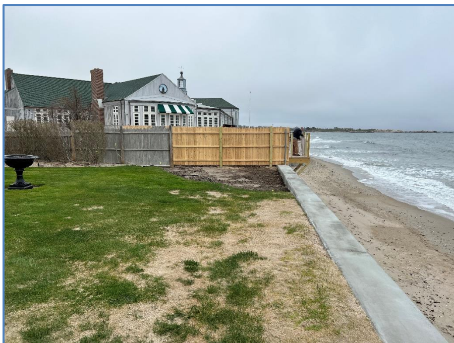
Figure 20: Upland behind Eastern Section of Seawall
