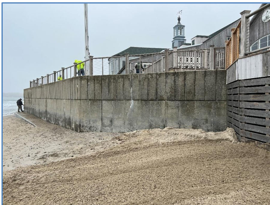
Figure 32: Return Section of Seawall
