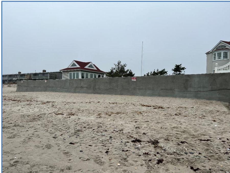
Figure 5: Western Side of Seawall
