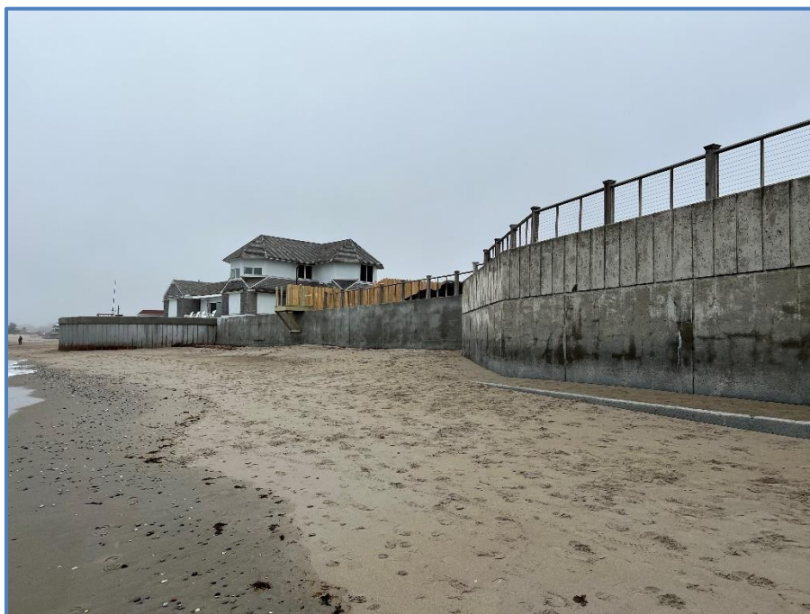
Figure 26: Concrete Seawalls Facing Northwest
