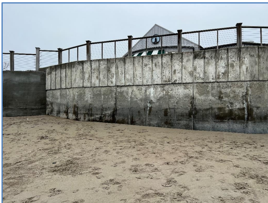
Figure 28: Start of Newer Section of Concrete Seawall
