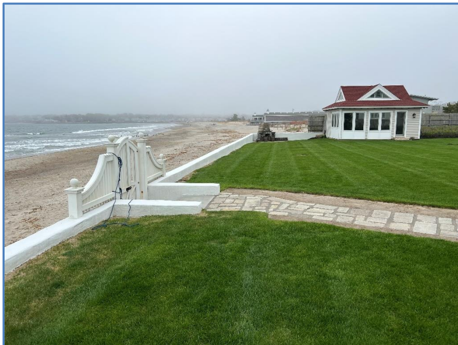
Figure 9: Upland Area Behind Western Side of Seawall
