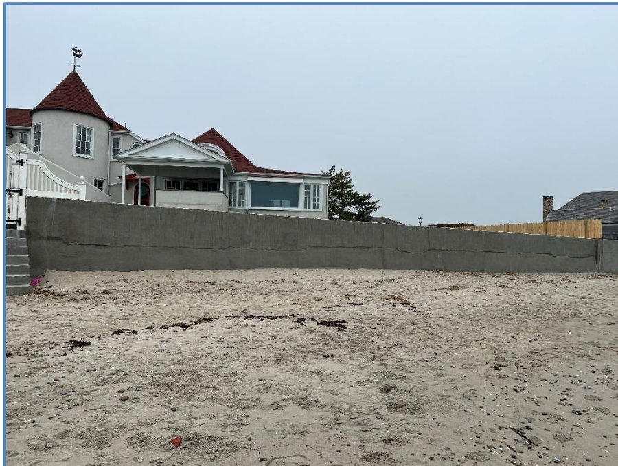
Figure 7: Eastern Side of Seawall
