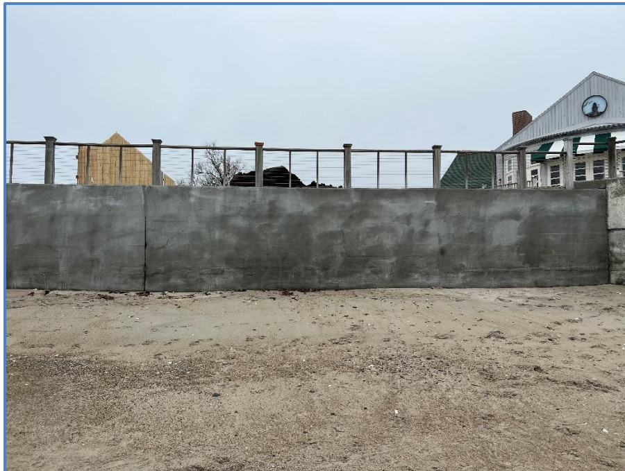
Figure 27: Older Section of Concrete Seawall
