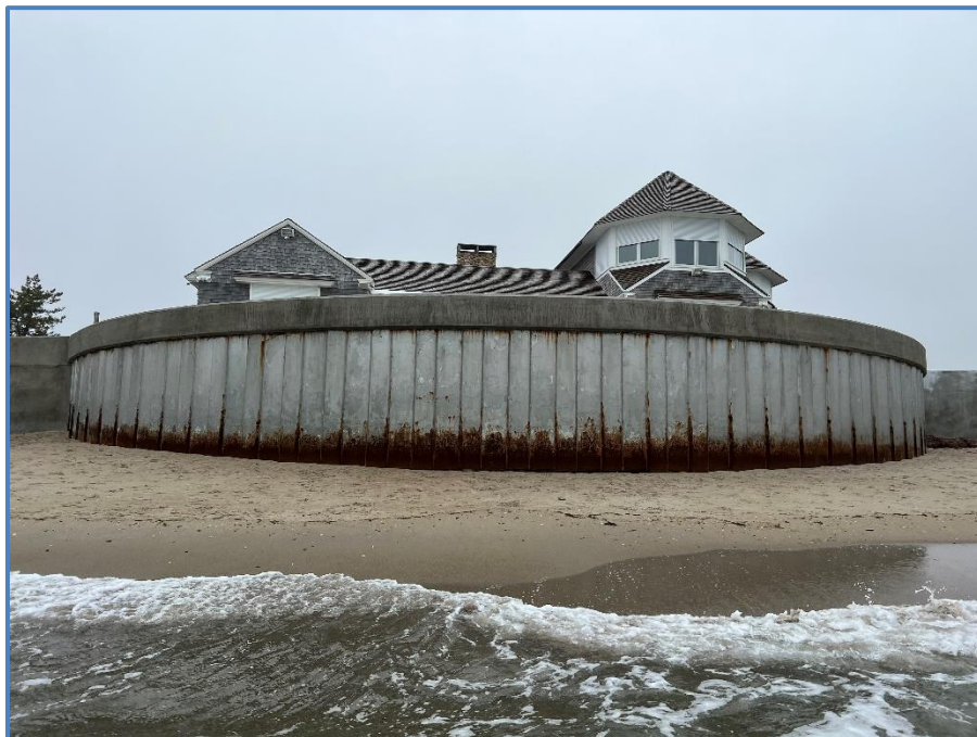
Figure 15: Middle Section with Curved Bulkhead
