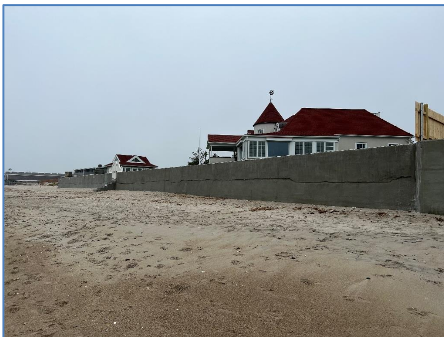
Figure 8: Seawall facing Southwest
