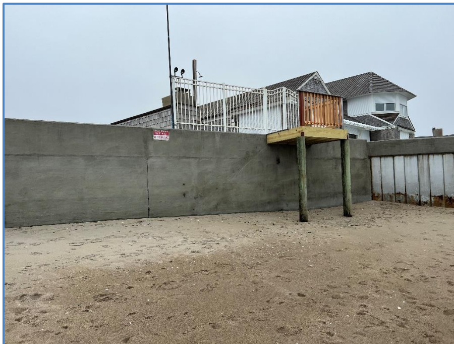
Figure 13: Western Section of Seawall and Access Stairs
