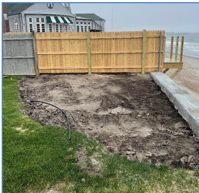
Figure 22: Area Restored From Undermining
