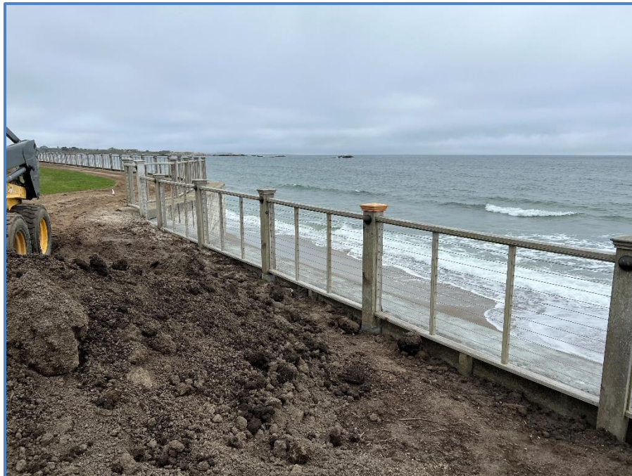
Figure 37: Upland Area at Older and Newer Sections of Seawall
