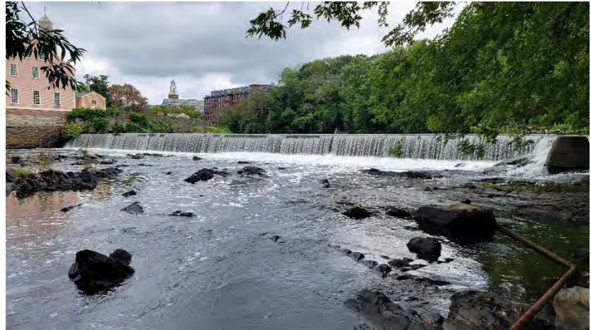
Illustration 2 – Northwest View of Slater Mill Dam
