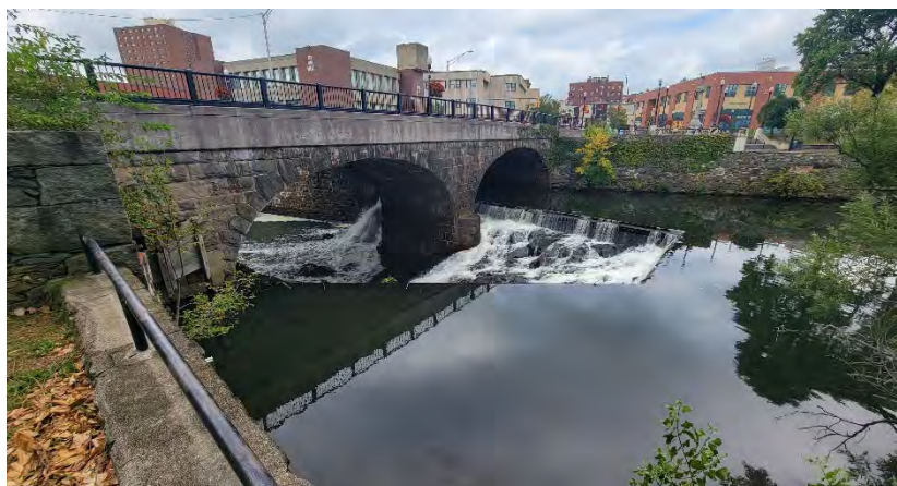
Illustration 1 – Southwest View of Main Street Dam
