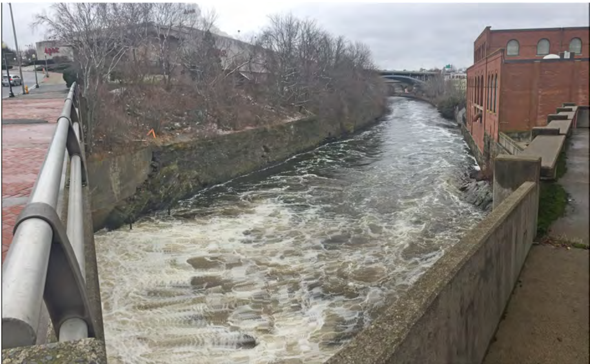
Overview of former Apex parcel riverbank facing downstream from Main Street bridge Main Street Bridge, facing south (February 2018)
