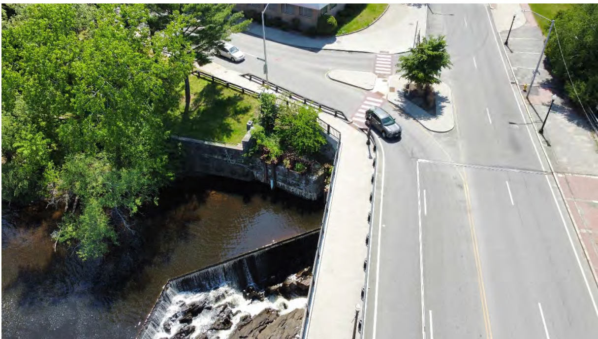
Aerial imagery of Slater Mill East Lot and Main Street Bridge, facing east (May 2021)
