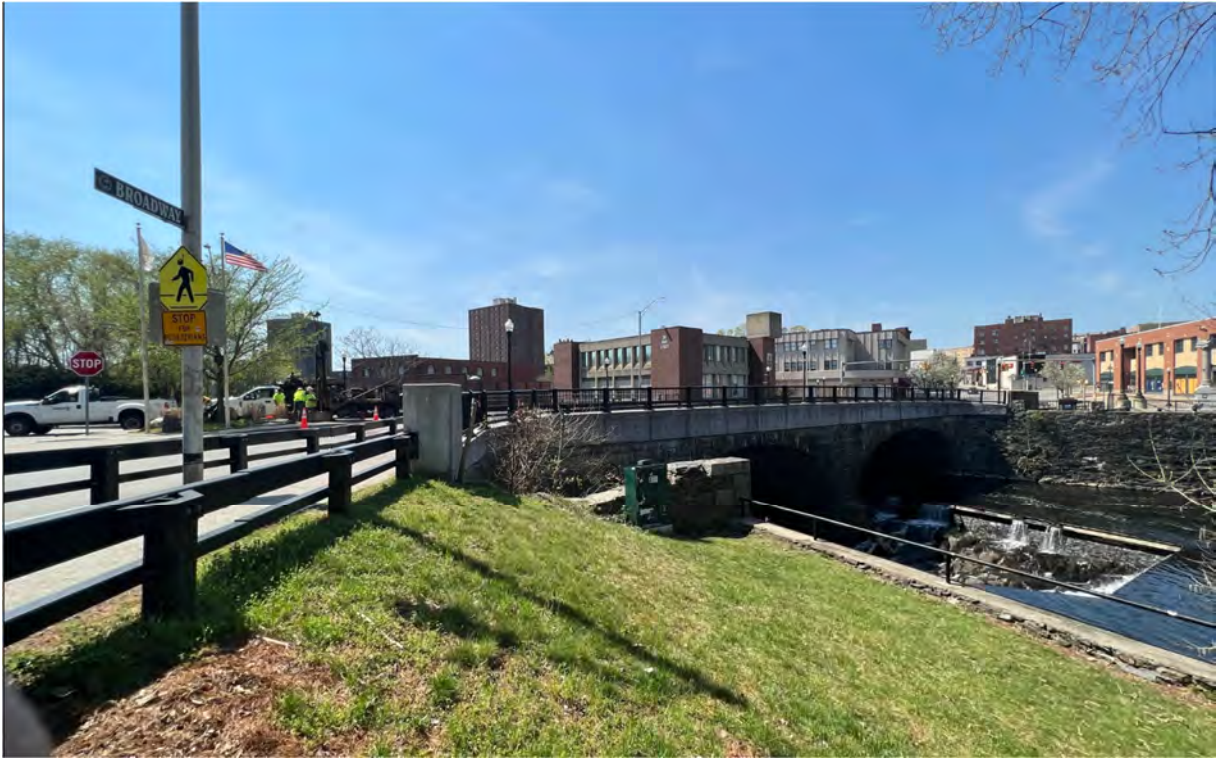
Main Street Dam and Bridge, electrical cabinet and vault (April 2021)
