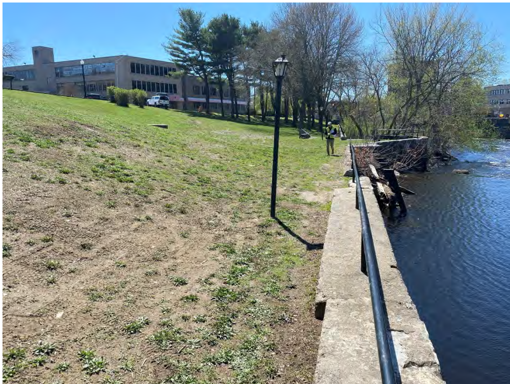
Slater Mill East Lot overview, facing south (April 2021)
