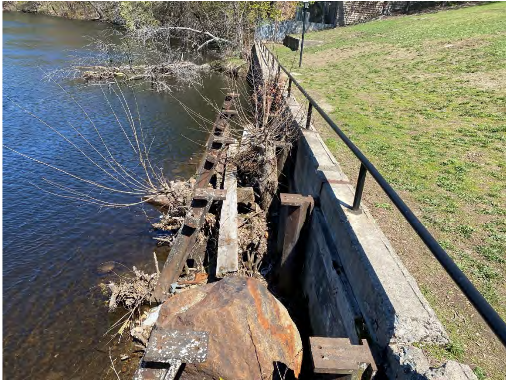
Former raceway intake gate remnant structures, facing north (April 2021)
