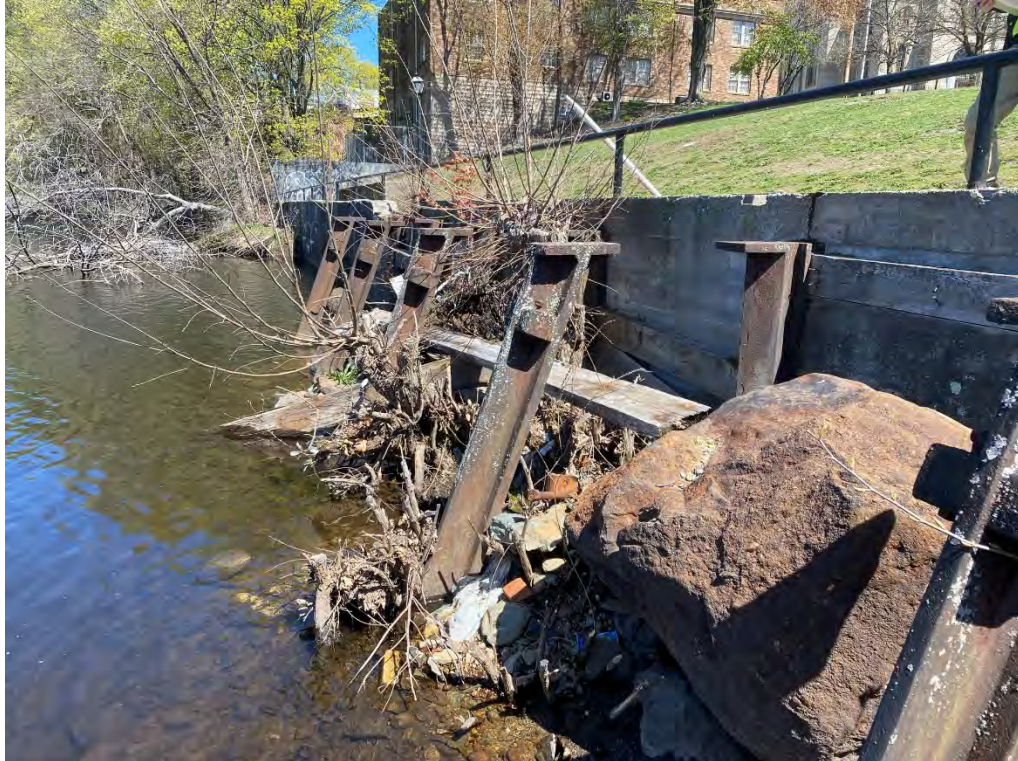
Photo 38: Concrete retaining wall, stop logs and entrained debris/boulder/sediment, facing north (April 2021)
