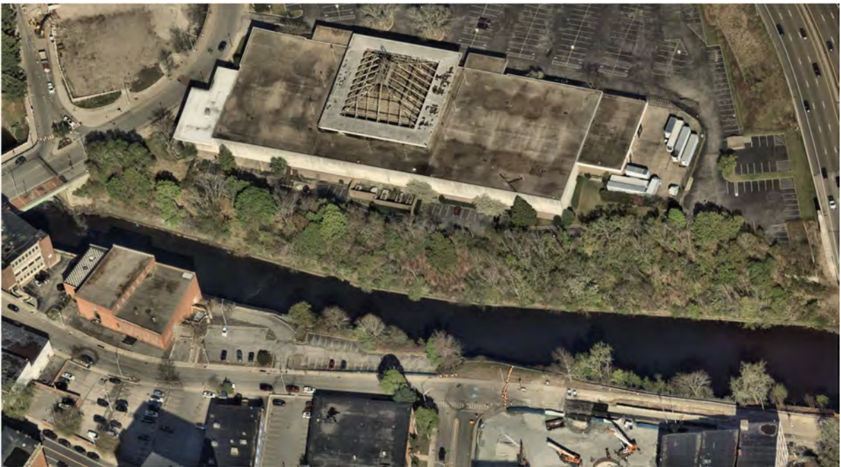
Aerial imagery of former Apex parcel, facing east (April 2025)
