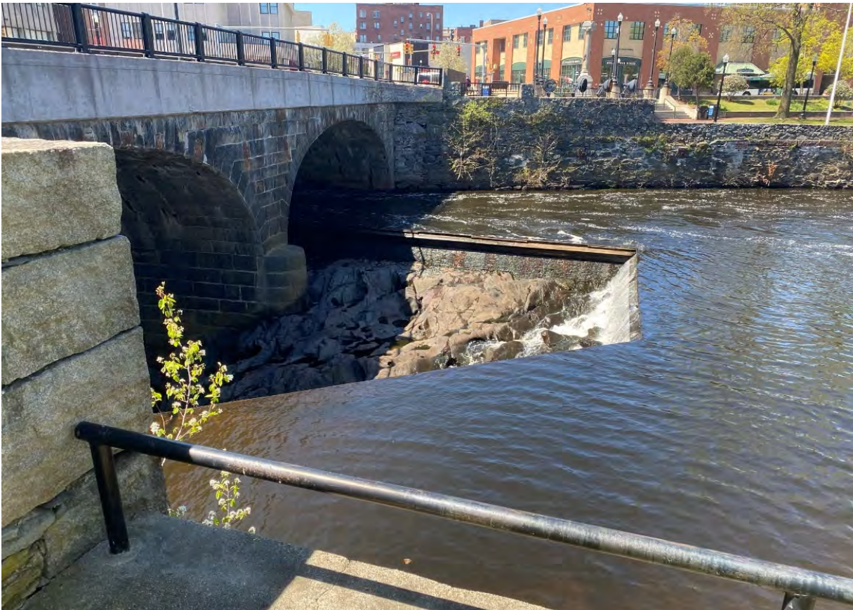
Main Street Dam, facing west (April 2021)
