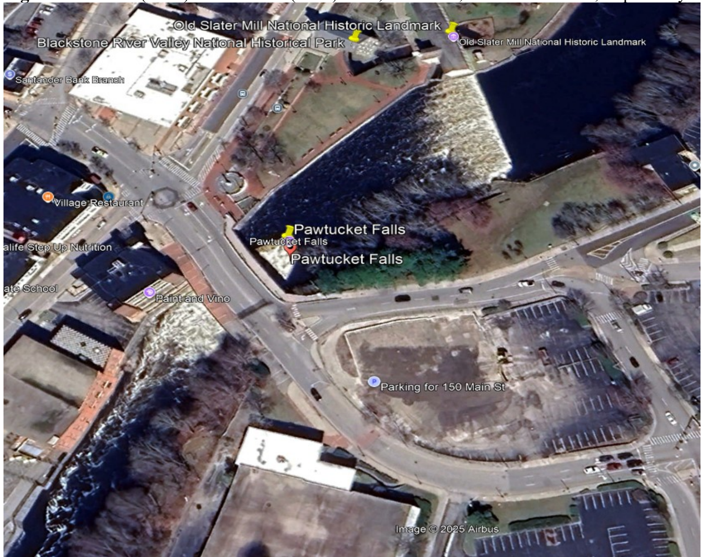
Figure 1: Main St (south) & Slater Mill (north) dams, Pawtucket, built 1896 & 1793, respectively
