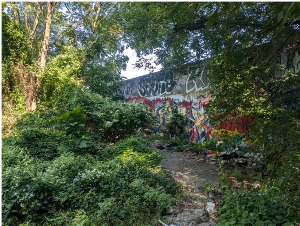
View of the large retaining wall at the northern extent of the Site that constitutes manmade shoreline—facing northeast.
