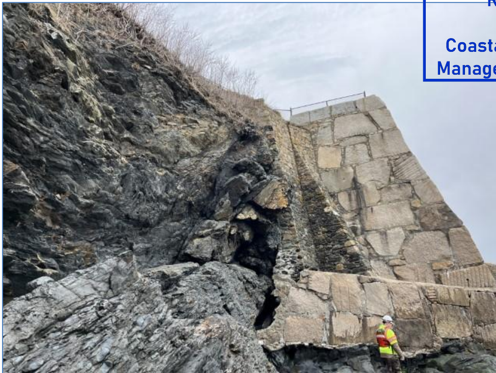
PHOTO 2: INTERWOVEN BEDROCK AT SECTION 1 CLIFF FACE - LOOKING NORTH
