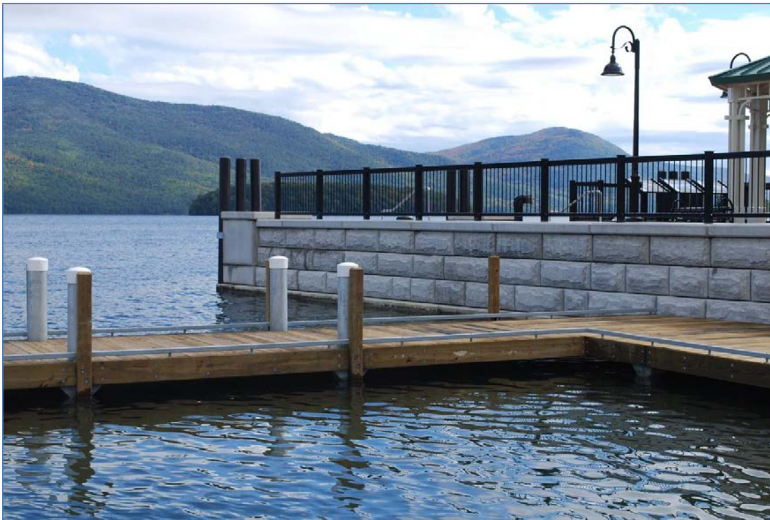
PHOTO 5: EXAMPLE PRECAST CONCRETE STONE STRONG SEAWALL (SOURCE – STONE STRONG)
