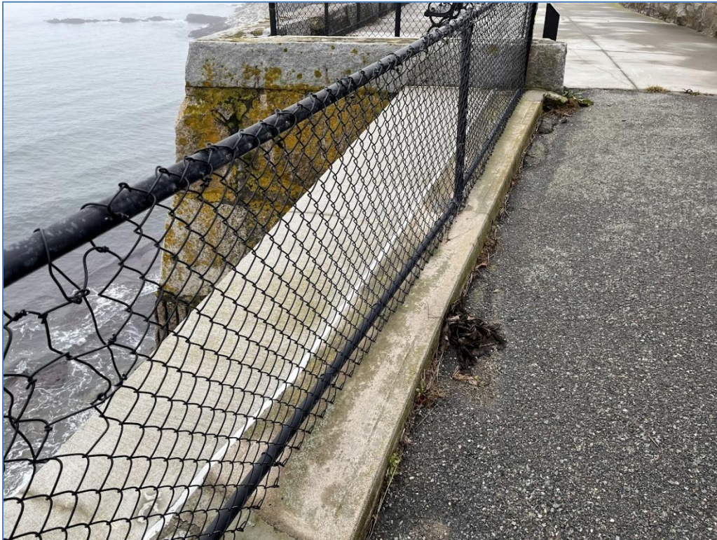
PHOTO 6: RAILING ALONGSIDE CLIFF WALK WITHIN PROJECT LIMITS
