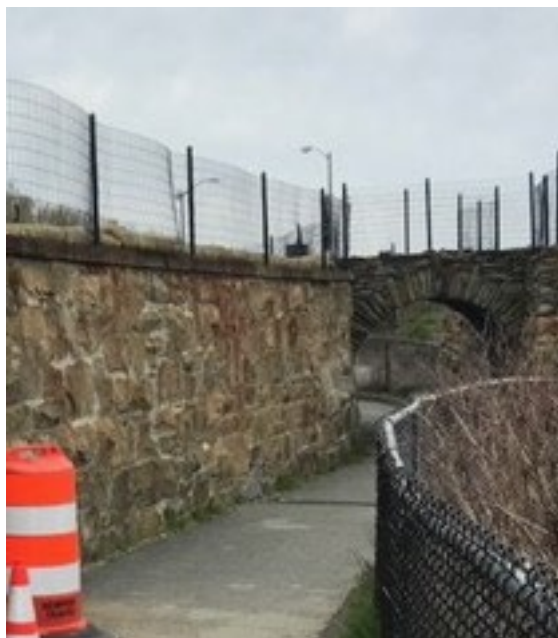
Photo 1: Stone Arch Bridge over the Cliff Walk walkway
