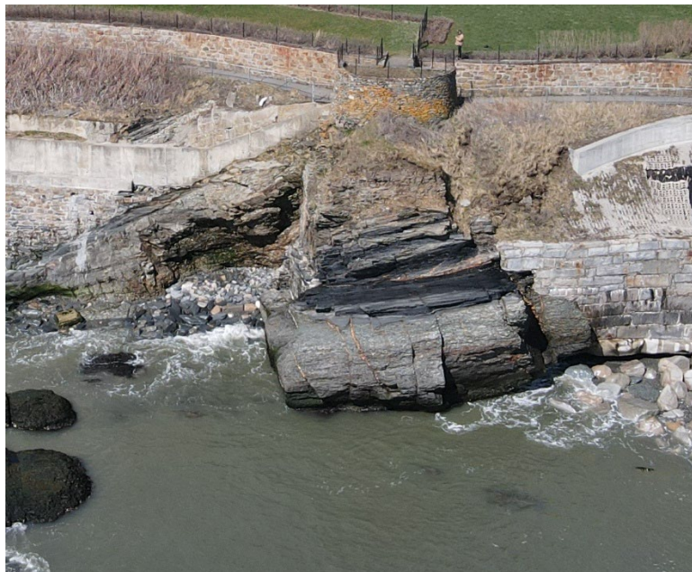
Photo 4: Overlook feature: note varying bedrock type along height – softer less competent rock up high
