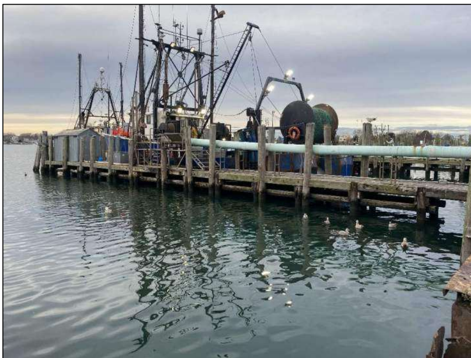
Photo No. 1.: View of Pier 'JJ' looking north.
