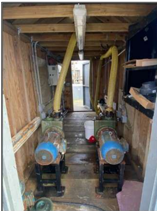
Photo No. 6.: View of the interior of the shed at the end of Pier 'JJ'.
