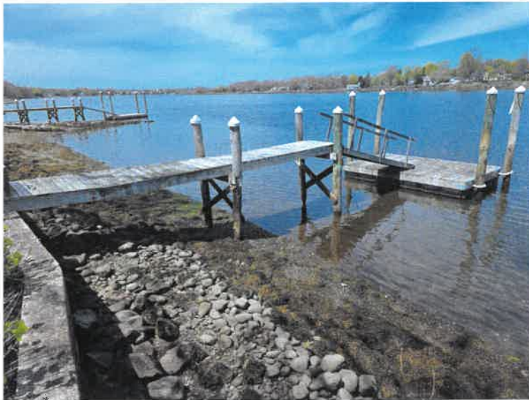
EXISTING FACILITY, LOOKING NORTH (2026)
