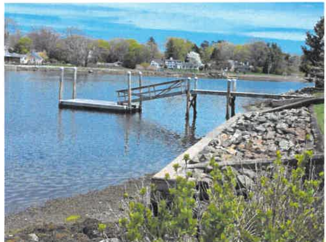
SOUTHERN ABUTTER, LOOKING SE (2026)
