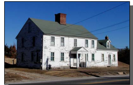
Reuben Mason House Restoration – Glocester
